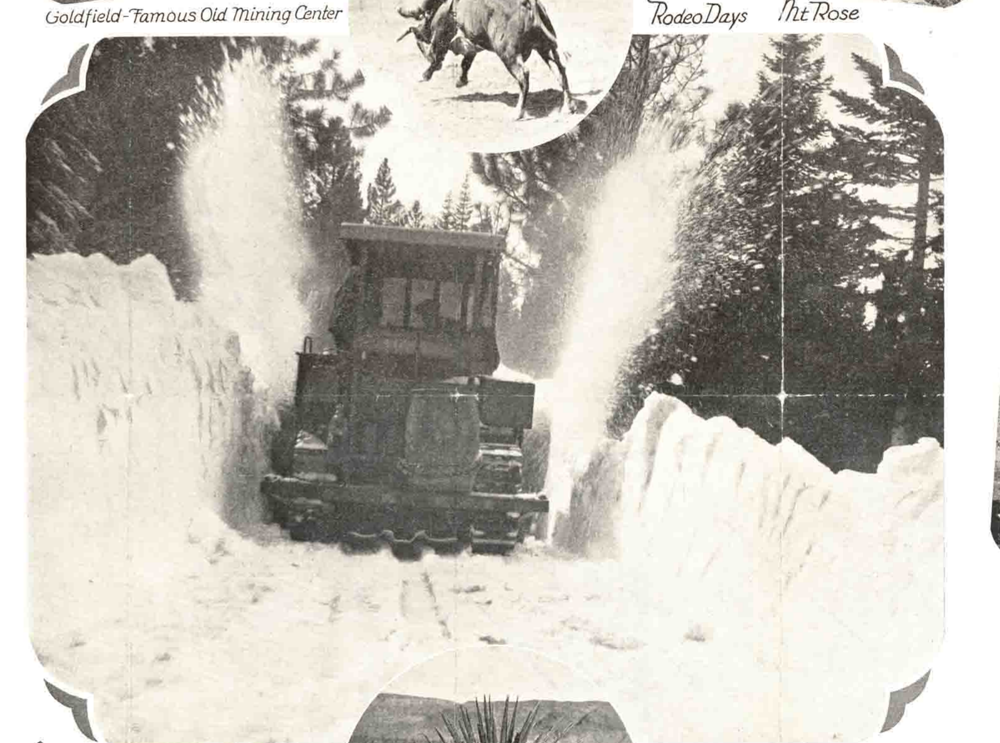
Snow Removal Equipment - Lake Tahoe
