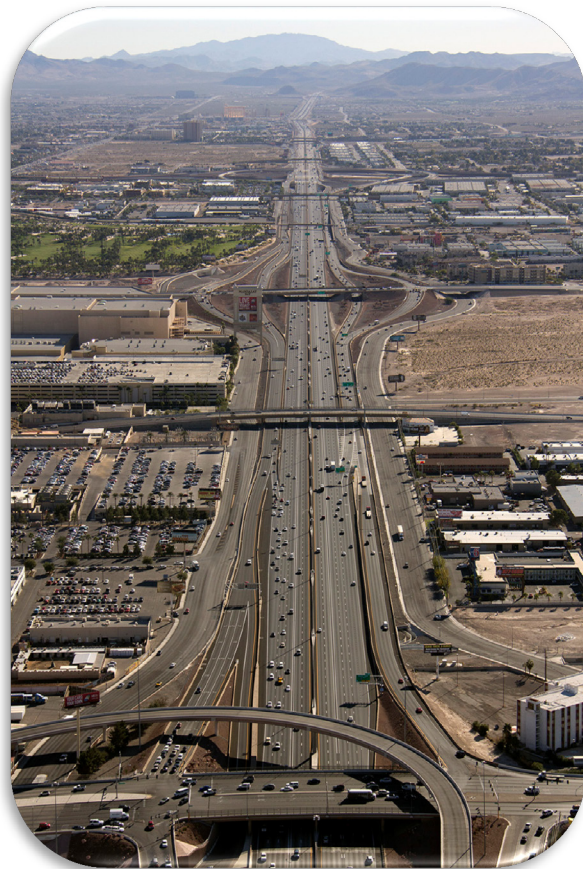
I-15 in Las Vegas (Interstate Freeway)
