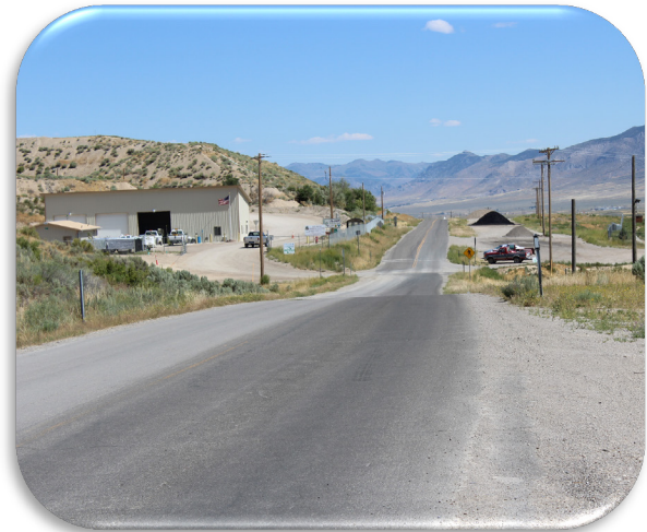
Lackawanna Road near Ely (Minor Collector)
