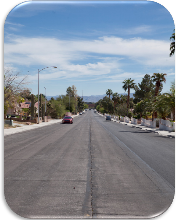
Eldorado Lane in Las Vegas (Frontage/Service/Local Road)
