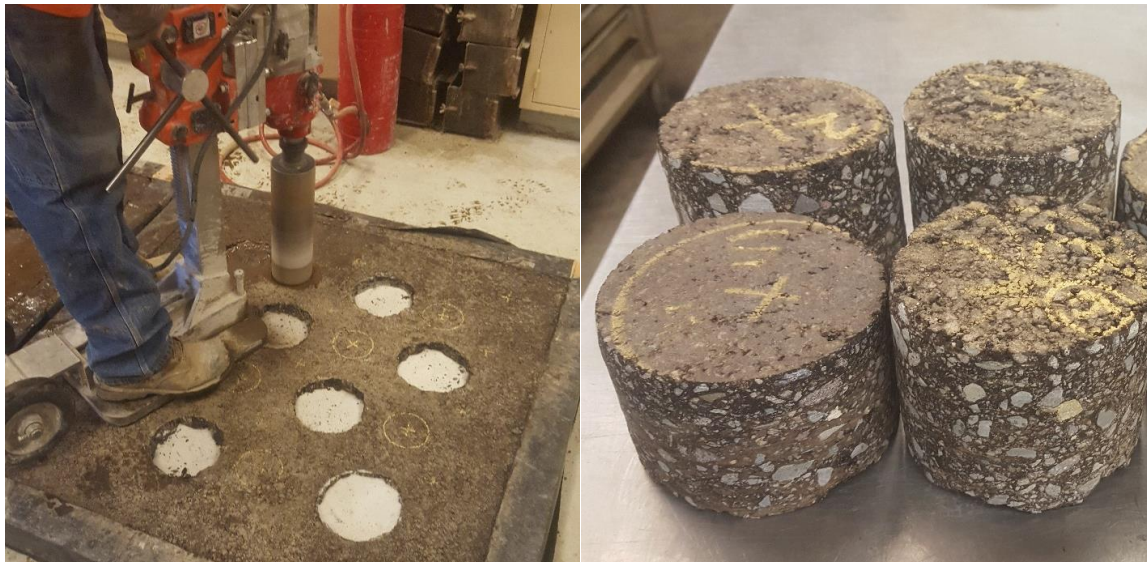
Figure 12. Coring of the CIR slabs.
