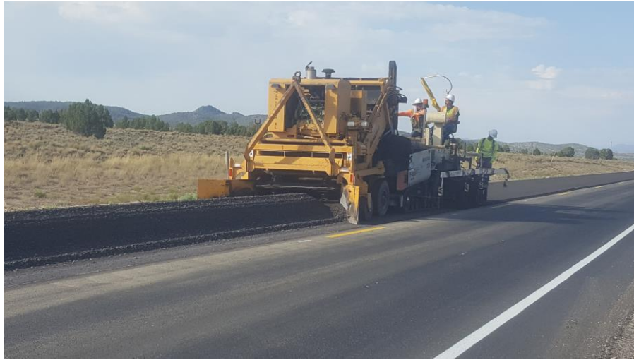
Figure 28. CIR construction on the Fernley CIR project.
