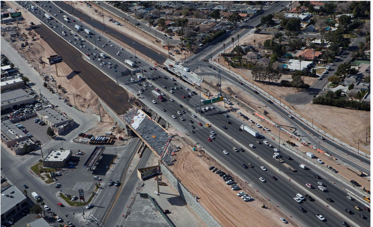
I-15 at Oakey Blvd Looking SE
