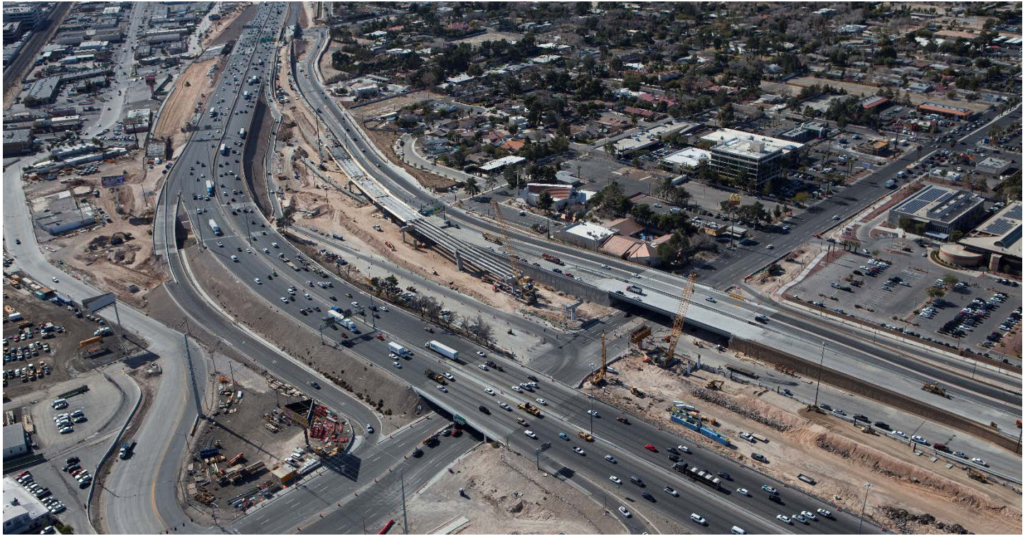
I-15 at Charleston Blvd Looking SE
