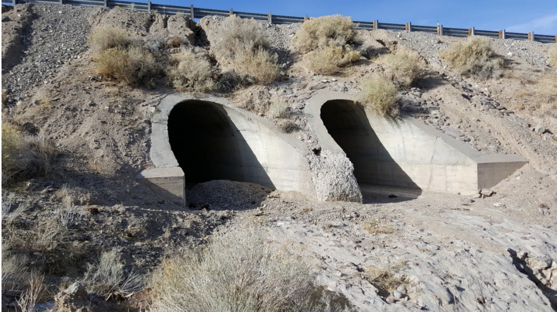
Double barrel concrete arch box. Photo looking west.
