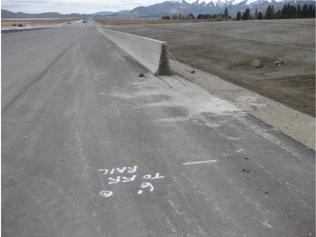
Barrier Rail Stakeout
