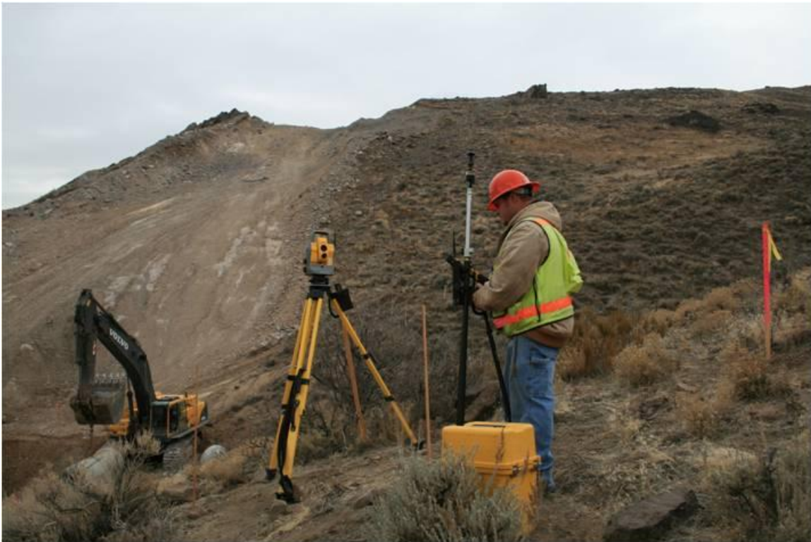
Trimble 5600 Robotic Total Station
