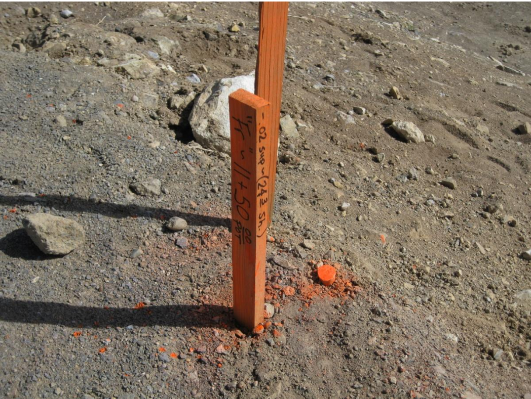
Slope Stake Showing Station, Superelevation, and Shoulder
