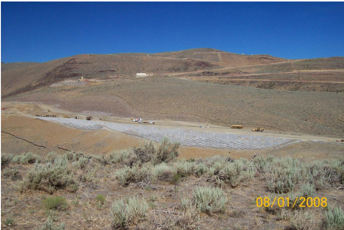
I-580 Freeway Under Construction
