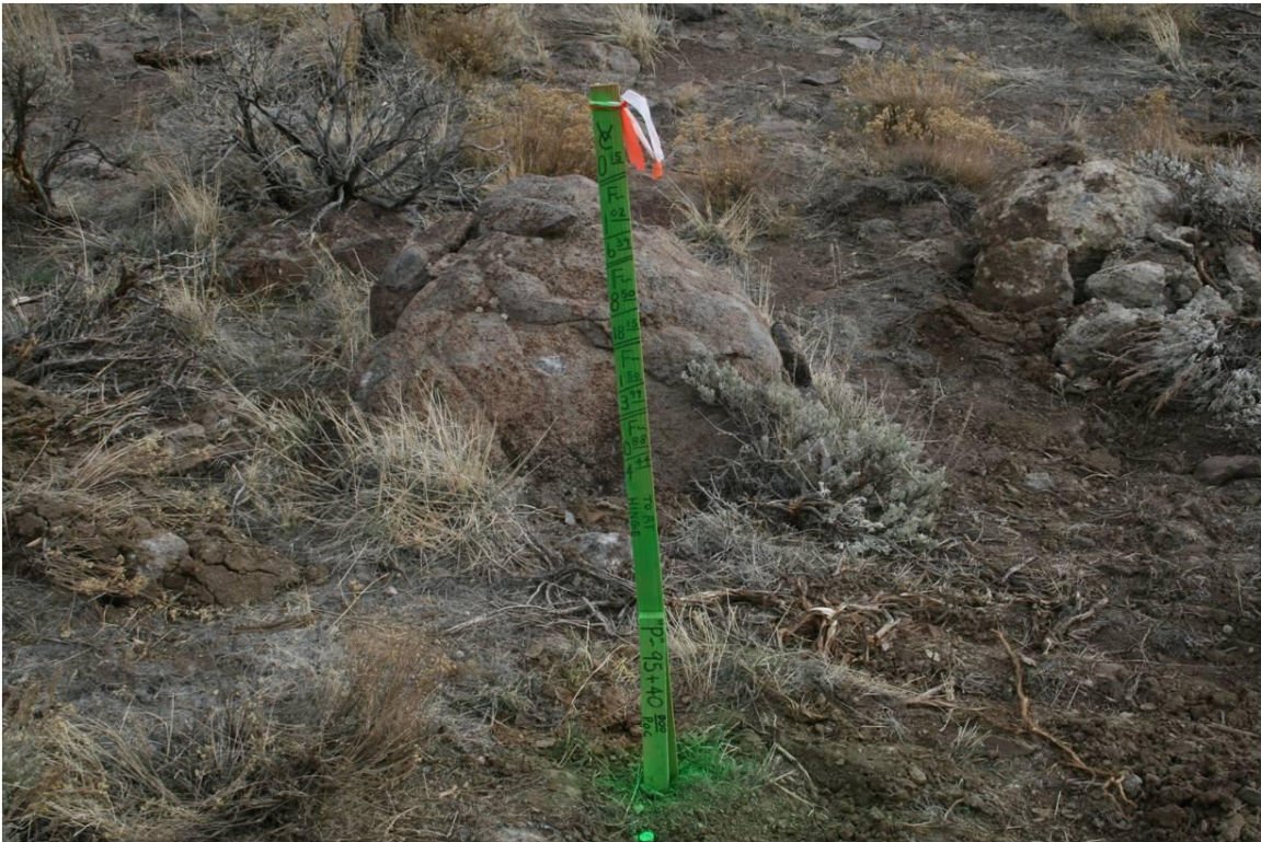
Slope Stake on the I-580 Project (Contract 3292)
