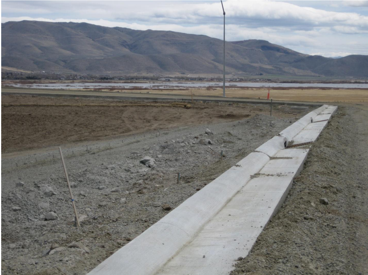
Curb and Gutter Stakeout
