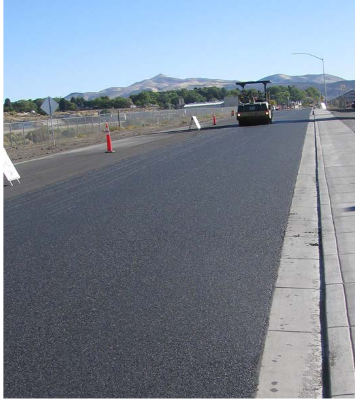
Figure 10 OGFC construction on SR 535.
