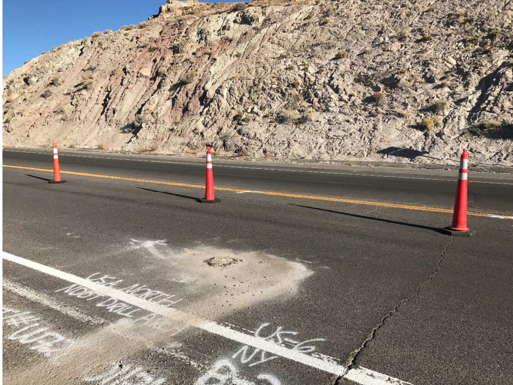
Boring US-6-NY-B-2 Location. Photo Looking East.
