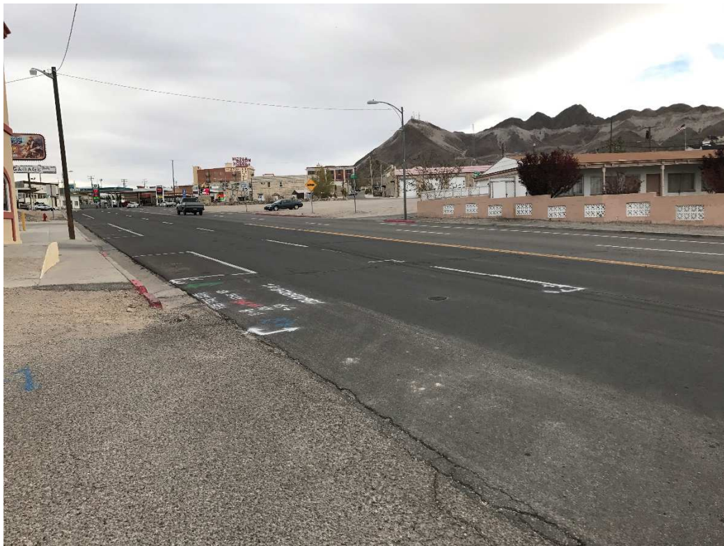
Boring US-6-NY-B-11 Location. Photo Looking South.
