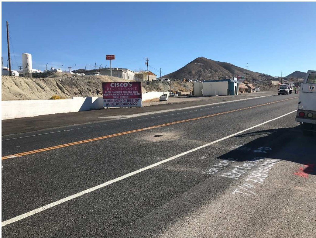
Boring US-6-NY-B-15 Location. Photo Looking South.
