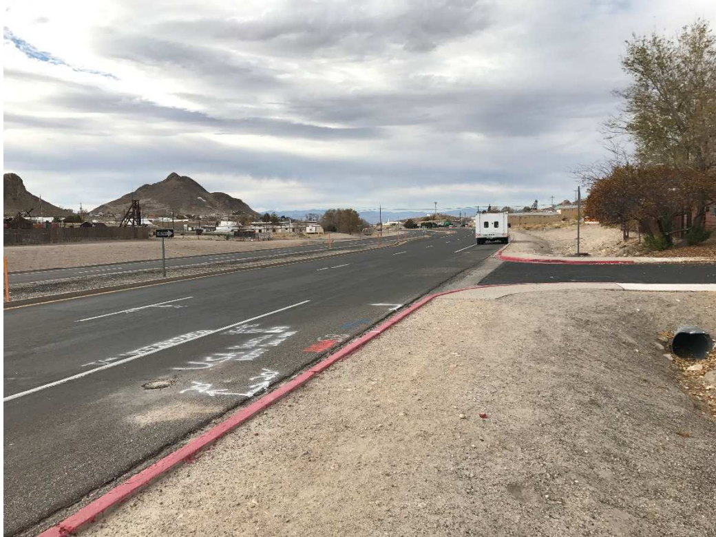
Boring US-95-NY-B-7 Location. Photo Looking North.
