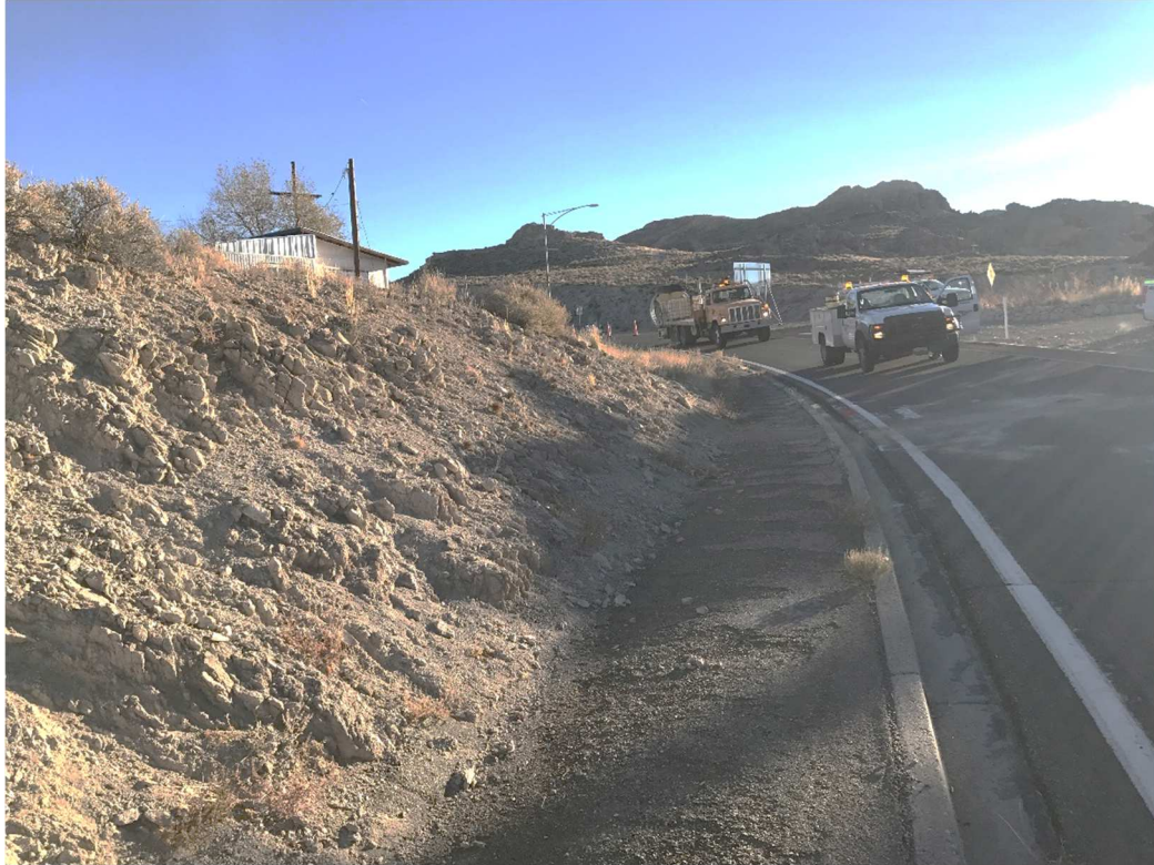
Boring US-6-NY-B-3 Location. Photo Looking East.
