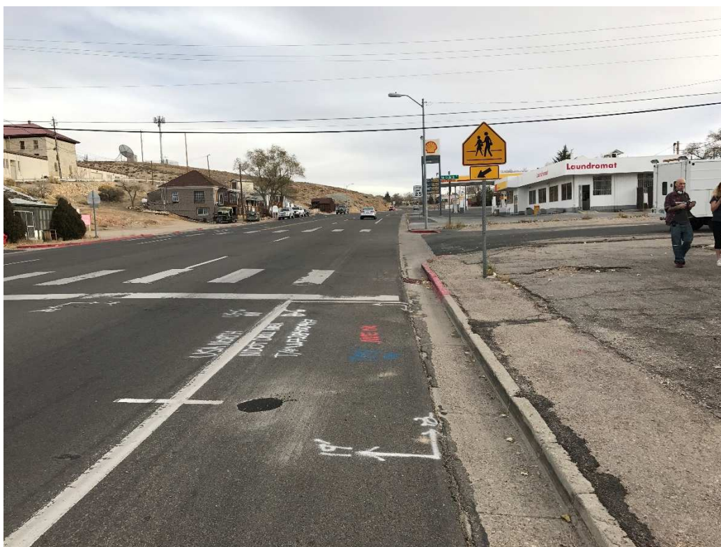
Boring US-6-NY-B-6 Location. Photo Looking South.
