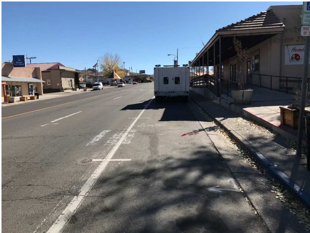
Boring US-6-NY-B-8 Location. Photo Looking South.
