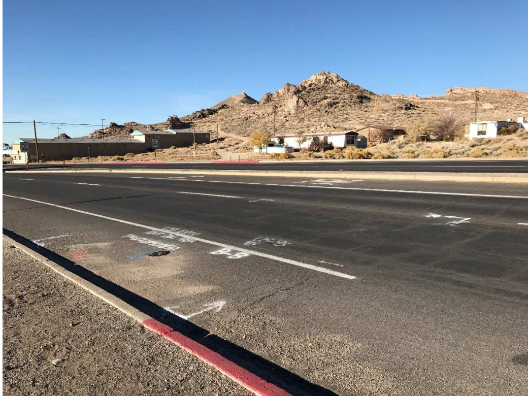
Boring US-95-NY-B-8 Location. Photo Looking Northwest.
