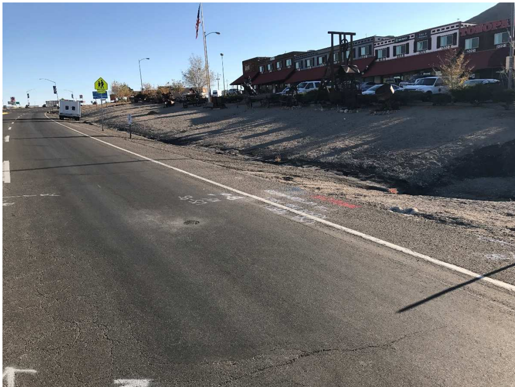
Boring US-95-NY-B-6 Location. Photo Looking South.
