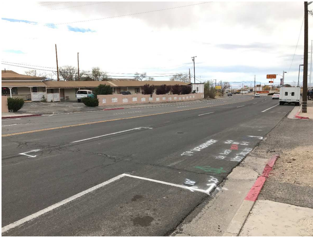
Boring US-6-NY-B-11 Location. Photo Looking North.
