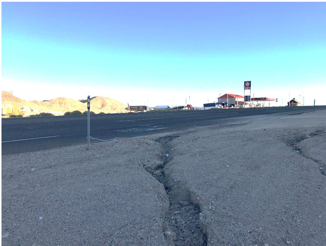
Boring US-95-NY-B-3 Location. Photo Looking South.
