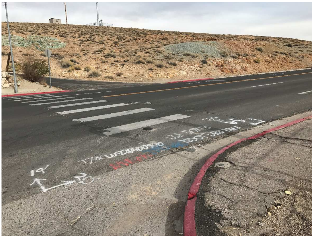
Boring US-6-NY-B-5 Location. Photo Looking East.
