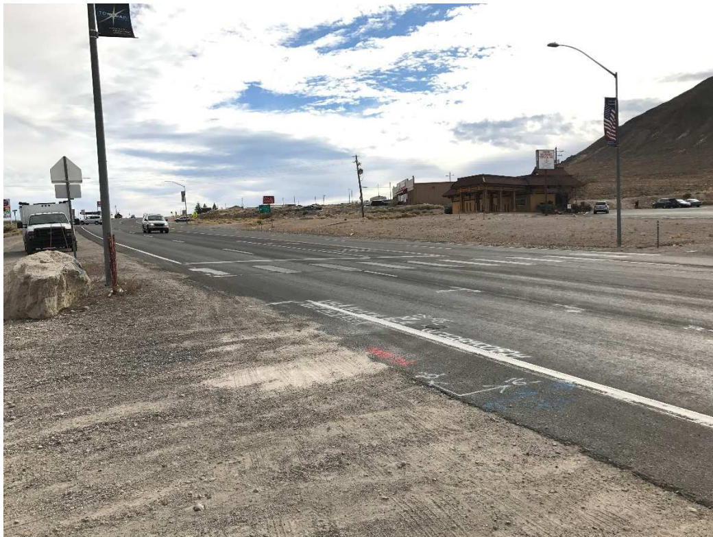
Boring US-95-NY-B-5 Location. Photo Looking South.
