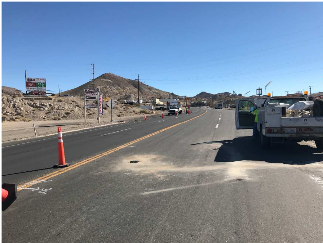
Boring US-6-NY-B-14 Location. Photo Looking South.
