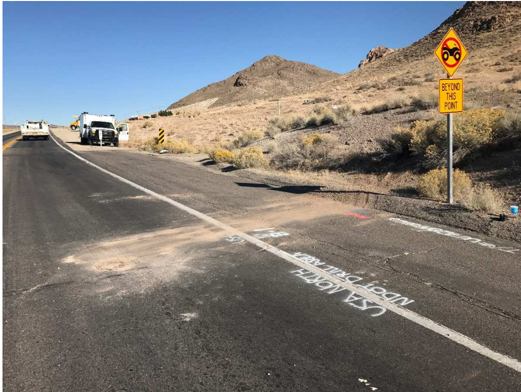
Boring US-6-NY-B-1 Location. Photo Looking East.
