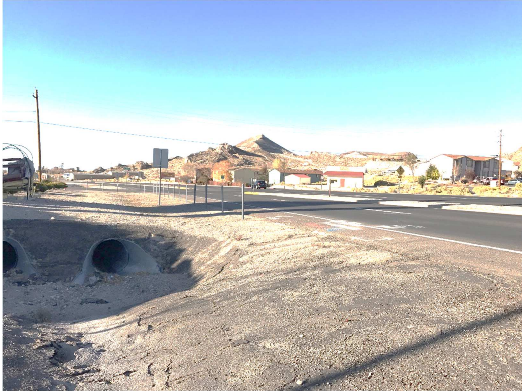
Boring US-95-NY-B-6 Location. Photo Looking North.
