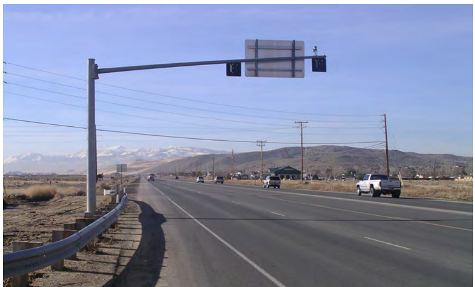
View of Study Area south of La Posada Drive looking south along Pyramid Highway
