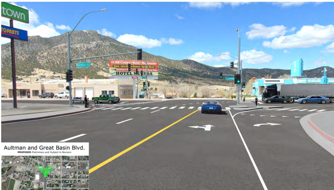
Aultman Street and Great Basin Boulevard - After Improvements
