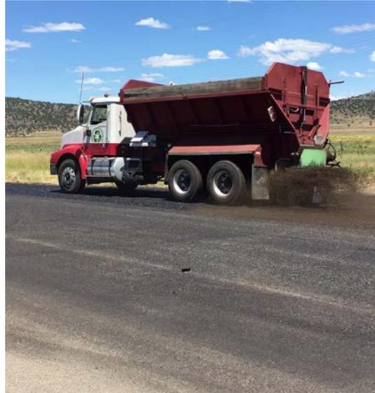
**Figure 4.6. Photo. Sand distributor during flush coat surface treatment application.**
