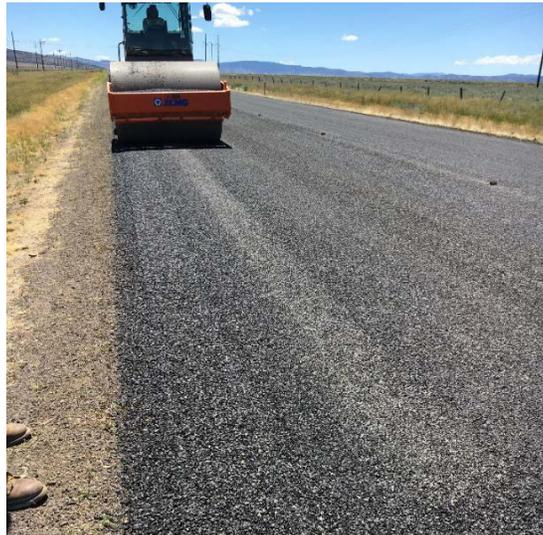
**Figure 4.5. Photo. Location of overlapped longitudinal joint after steel drum roller.**
