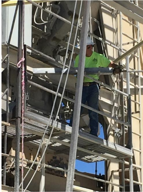
**Figure 4.8. Photo. Hot bin 3/8 inch chip sampling.**
