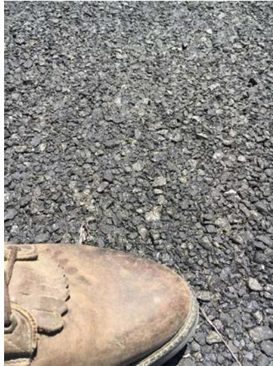
**Figure 4.4. Photo. Chip seal surface upon completion of rolling operations.**
