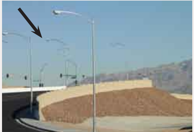
(1) Not Recommended: Over-Lighting Roadway Facilities.
