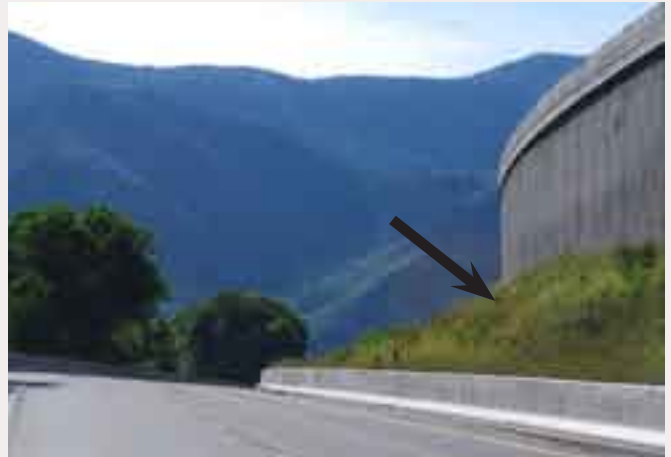
(1) Recommended: Using Landform and Grading to Reduce Wall Height and Open Views.
