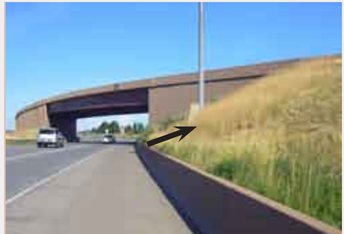
(1) Recommended: A Revegetated Embankment Slope.
