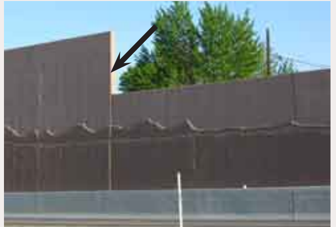
(1) Not Recommended: Disproportionate Wall Height Transition.
