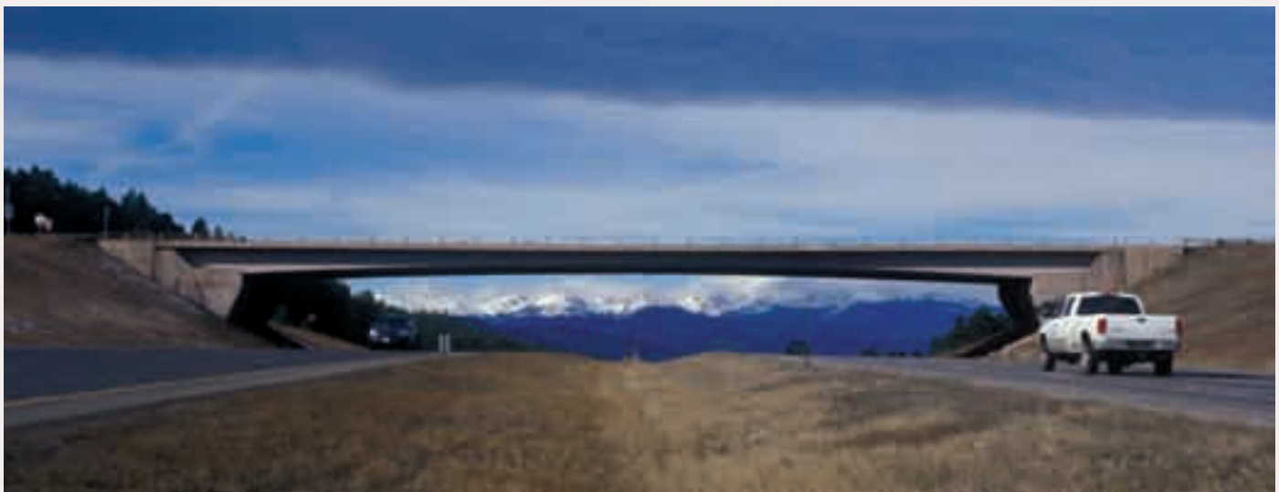
(1) This bridge is visually appealing because it relates to the site and views. The proportion of its form and mass are appropriate - the abutments appear to be sized to perform their function in relation to the superstructure.
