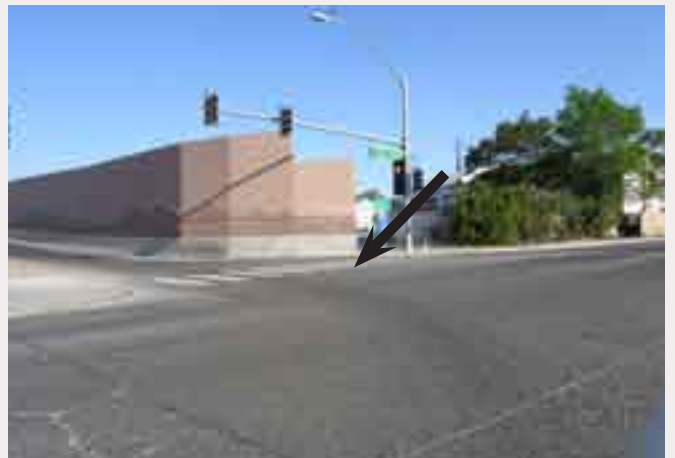
(2) Not Recommended: Abrupt Termination of Sound Wall.
