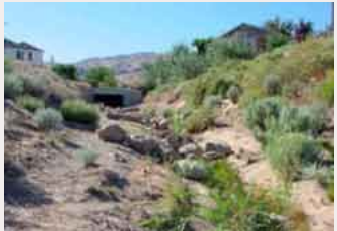
(1) Recommended: Revegetated Drainage Channel.
