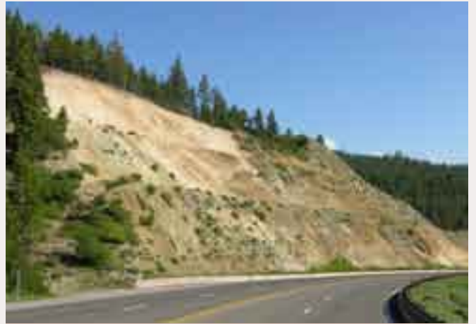
(1) These steep cuts and benching visually scar the landscape and are difficult to revegetate in Nevada's arid climate.
