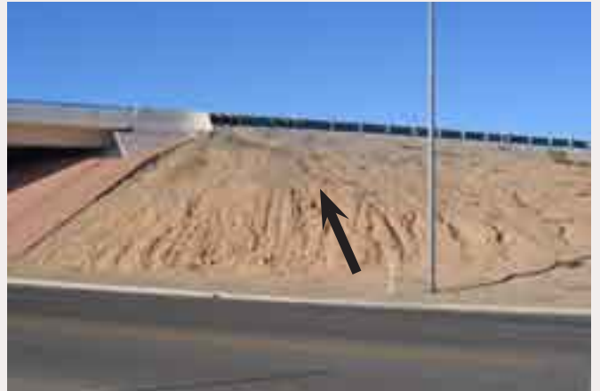
(1) Not Recommended: A 2H:1V Slope.
