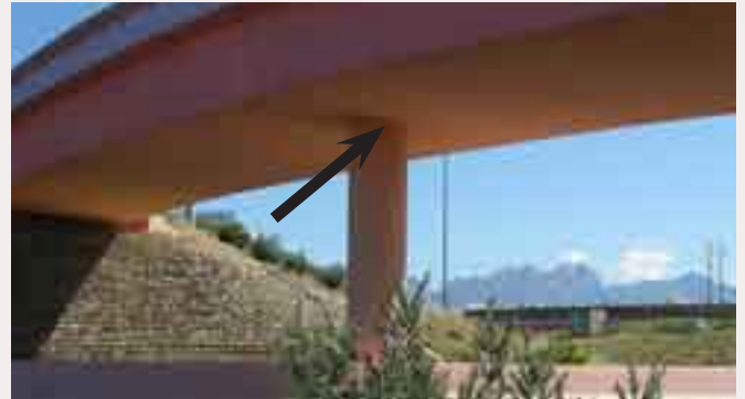
(1) Recommended: Integral Pier Cap.
