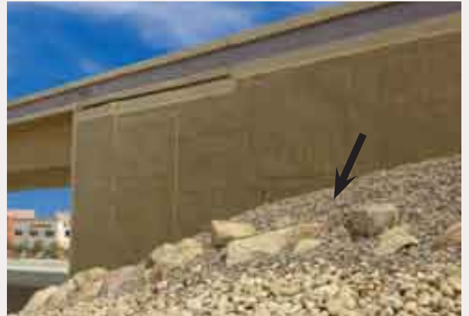
(1) Recommended: Rock Mulch Embankment Slope.
