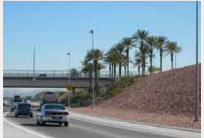
(1) In southern Nevada, large quantities of rock mulch are used to stabilize slopes and provide dust and weed control. The overuse of rock mulch eliminates the potential for slope revegetation and a softening of the highway environment.
