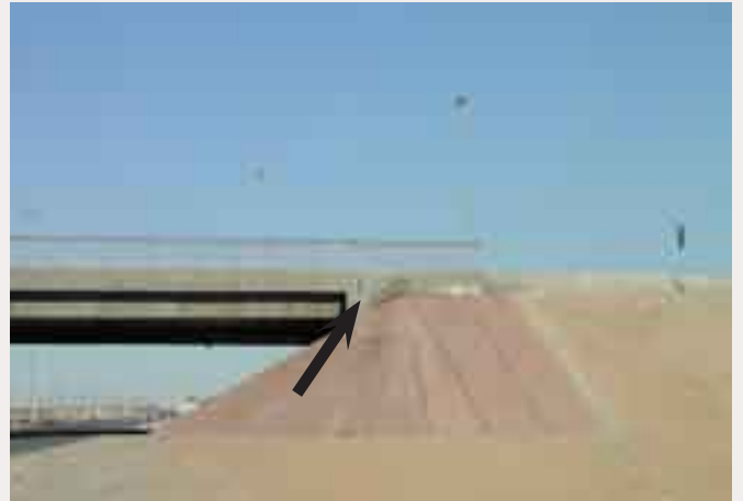
(1) Not Recommended: Abutment exposure of 2' or less.
