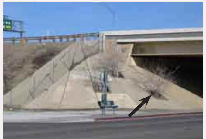
(2) Not Recommended: Tree Wells in Slope Paving.
