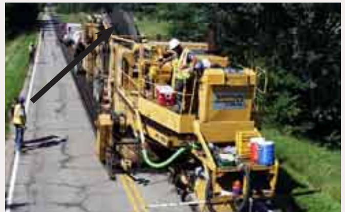
(2) Recommended: Recycling Cold Millings for Paving Overlays.
