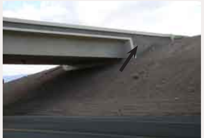
(2) Not Recommended: Abutment exposure of 2' or less.
