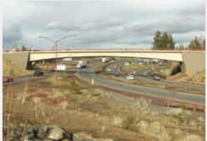
(1) The goal of highway design is to satisfy safety, environmental, structural, and visual needs in order to create site appropriate design solutions.
