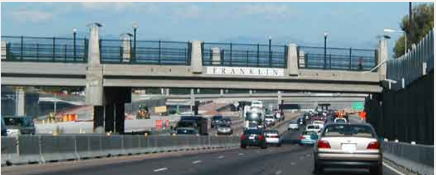
(2) As seen here, in busy traffic conditions, straight-forward aesthetics that increase wayfinding and the motorist's ability to navigate the highway system are preferred over other attention-grabbing designs.
