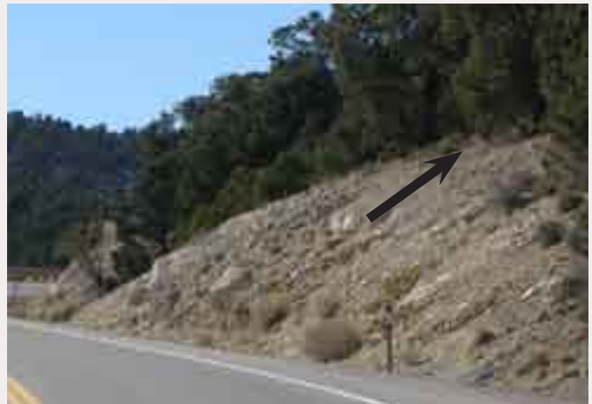
(1) Recommended: Slope Rounding.
