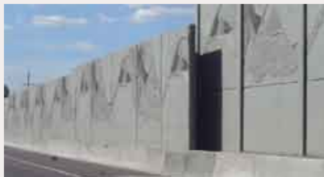
(1) Sound walls should be thoughtfully coordinated with the barrier rail as shown above.
