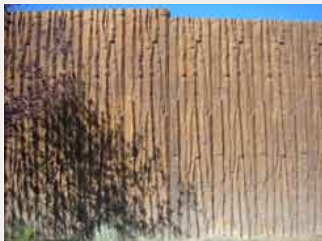
(2) Sound walls provide a great opportunity to reflect the surrounding context through aesthetic patterning.
