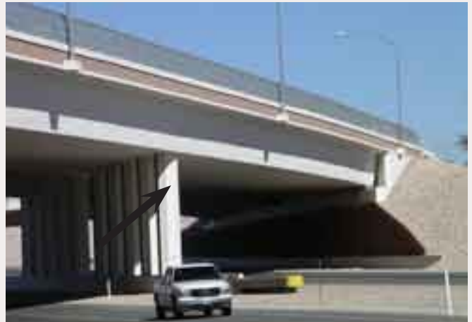
(2) Not Recommended: Use of Numerous, Small Diameter Piers.
