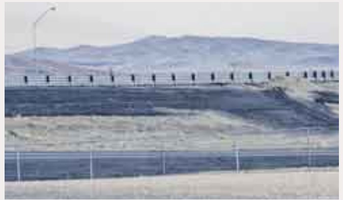
(1) Coldmillings have negative visual impact. Distinctive black bands are visually distracting and unattractive.
