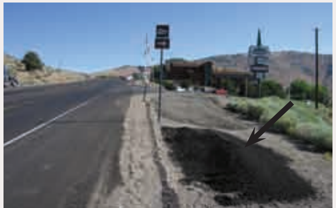
(3) Not Recommended: Piling Millings Along Shoulder.
