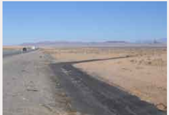
(2) Lining roadside swales with asphalt increases water velocity and the intensified flows can lead to increased downstream erosion and stabilization issues. Another negative element is the way it visually stands out against the landscape.
