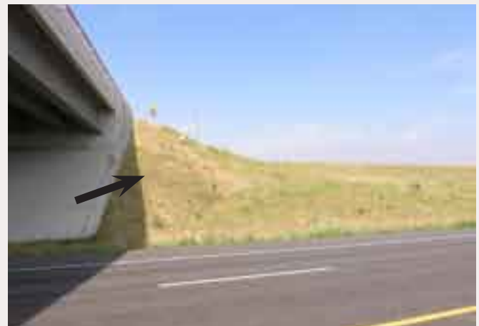
(2) Recommended: A Revegetated Embankment Slope.
