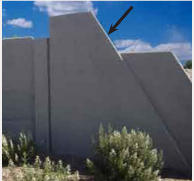
(1) Recommended: Wall End Piece Transitions Between Top of Wall and Barrier Rail.
