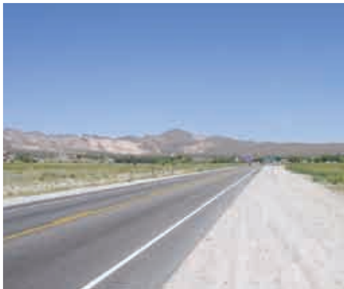
(2) The existing shoulders may not be adequate for heavy truck traffic with hazardous waste.
