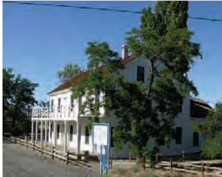
(3) Historic buildings provide opportunities for rest areas and interpretive features.
