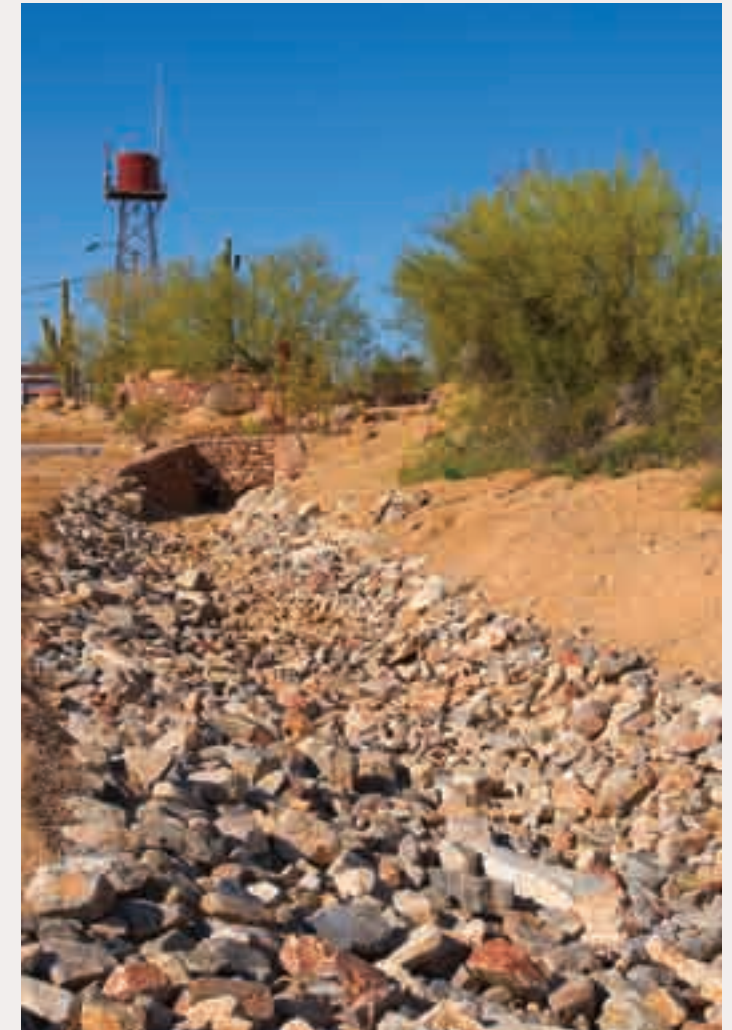
(1) Rock ground treatments should harmonize with existing soils. Aesthetic placement integrates drainage systems as part of the design. Water can be directed to cisterns for storage and later use.
