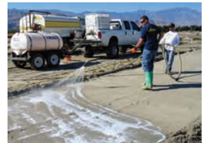
(2) Application of soil stabilizer aids in dust and erosion control.
