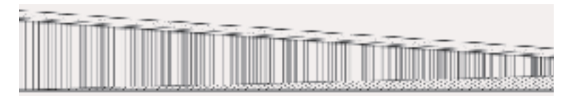
(10) Preferred finish is rusticated variable vertical texture and pattern. Surfaces should have a single finish whether MSE, cast-in-place, or other wall type is used. Consistency with other structures is required.
