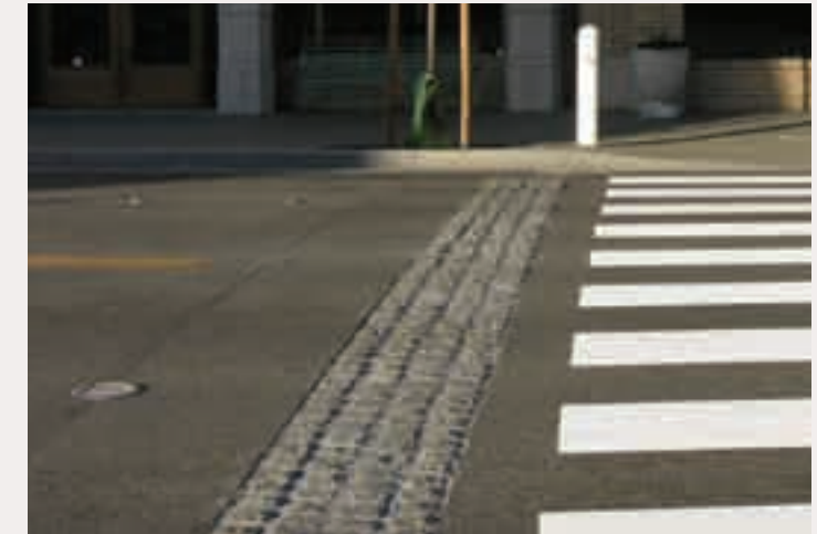
(2) Flashing pedestrian crossing signals enhance pedestrian visibility by motorists. In the above image, sensors on either side of the crosswalk activate flashing lights in the pavement when pedestrians cross the street.
