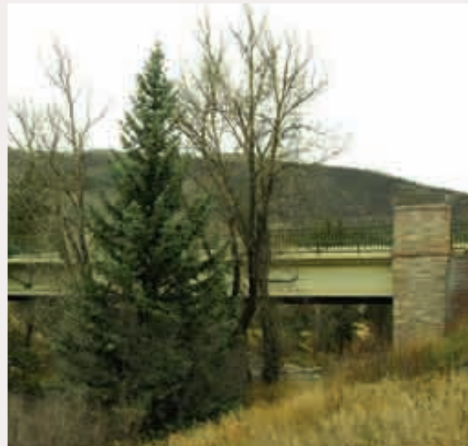
(12) Bridge forms should be simple and abutments should visually support the structure.
