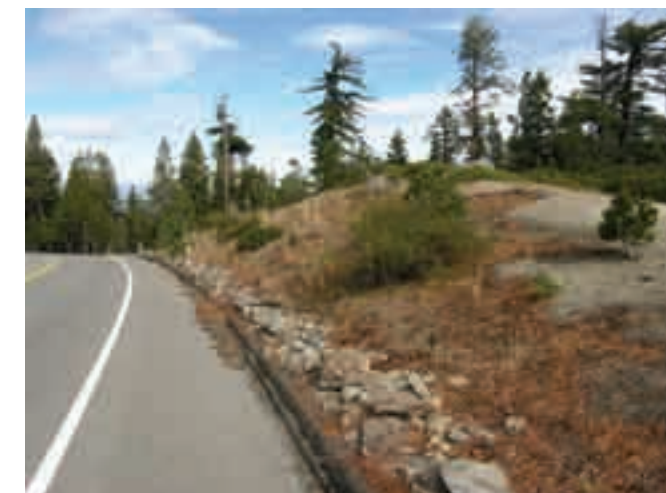
(1) Native rock and vegetation add aesthetic value while stabilizing slopes.
