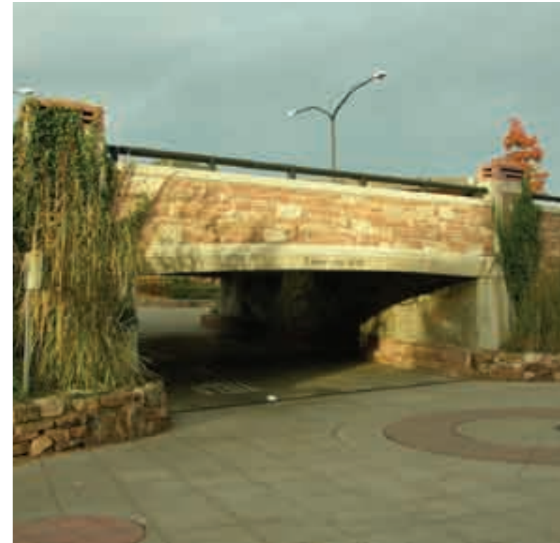
(1) The length of underpasses should be minimized where possible in order to allow natural lighting.
