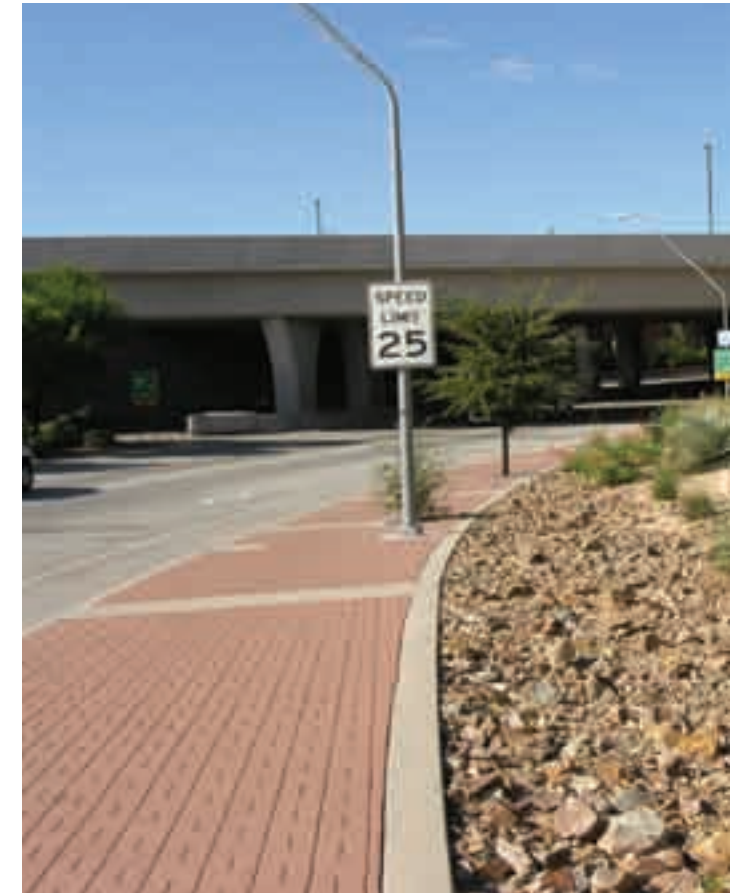
(1) Landscapes require varying degrees of upkeep and should be designed with an understanding of the long-term maintenance implications.
