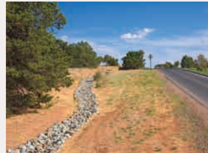
(1) Rock-lined drainage channels are an attractive alternative to concrete or unlined ditches.
