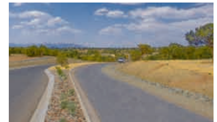
(4) Rock lined medians, alone or in combination with drainage swales, allow for runoff of excess stormwater.
