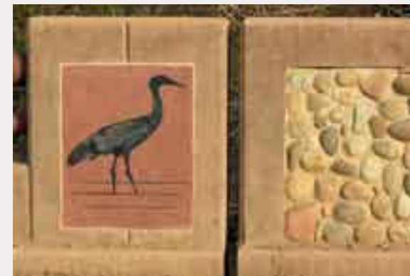
(7) Art incorporated into bridges and structures subtly invoke special meaning.
