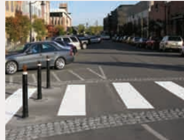
(1) Zebra striped crossings require less maintenance and are more noticeable than standard parallel striping.
