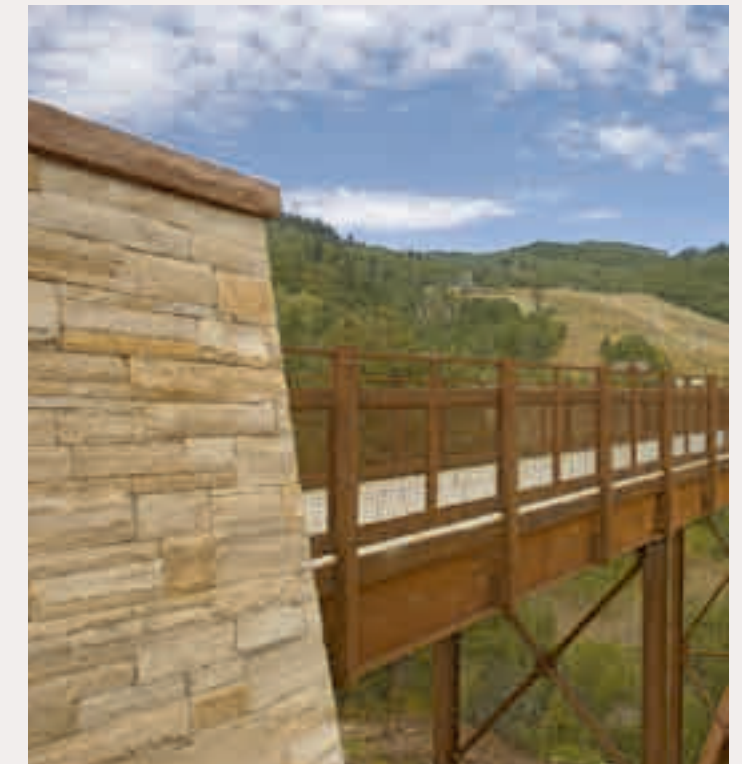
(15) Subtle bridge materials enhance place-making and add visual interest.
