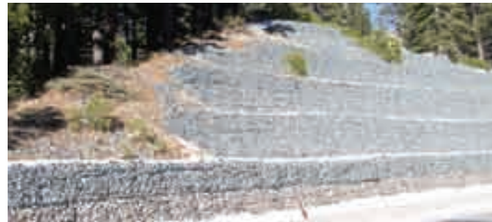
(8) Avoid gabion retaining walls that utilize large light-colored rocks. Narrow spaces between terraces prevent the ability to plant native vegetation for visual relief.
