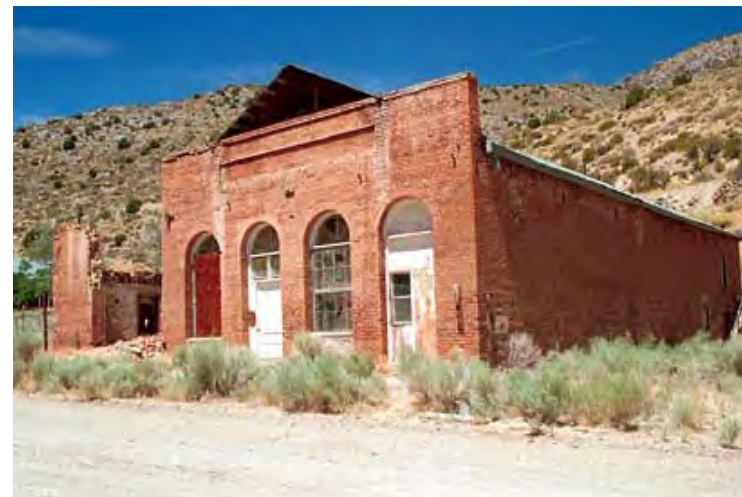
(3) The history of abandoned mining towns across the state provides a unique interpretive opportunity.
