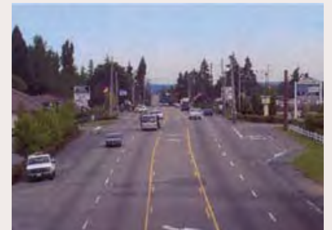
(2) Before streetscape improvements.
