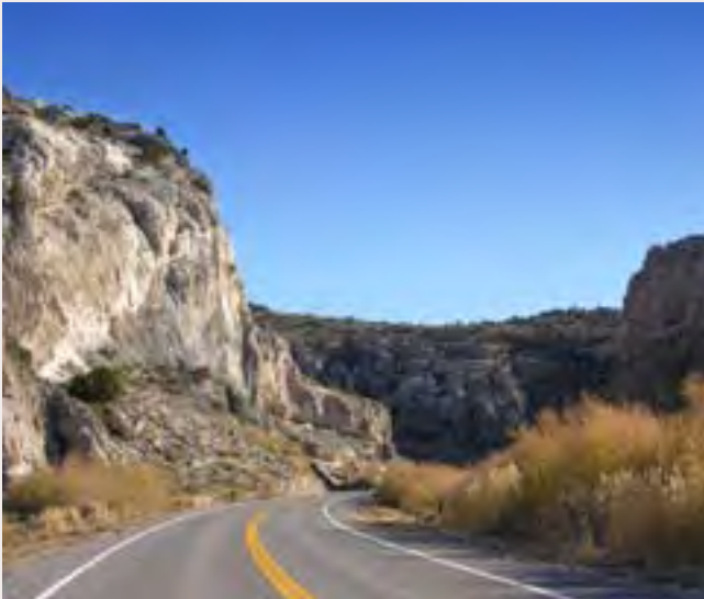
(2) Maintaining an undisturbed right-of-way is the prime focus for the Silver State Passage segment. Revegetation uses native plants that fit within the surrounding plant community.
