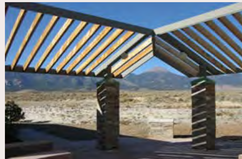
(3) Nevada's harsh arid climate mandates shelter from the wind and sun be provided at all rest areas. Structures should provide travelers shelter without detracting from the overall surroundings.
