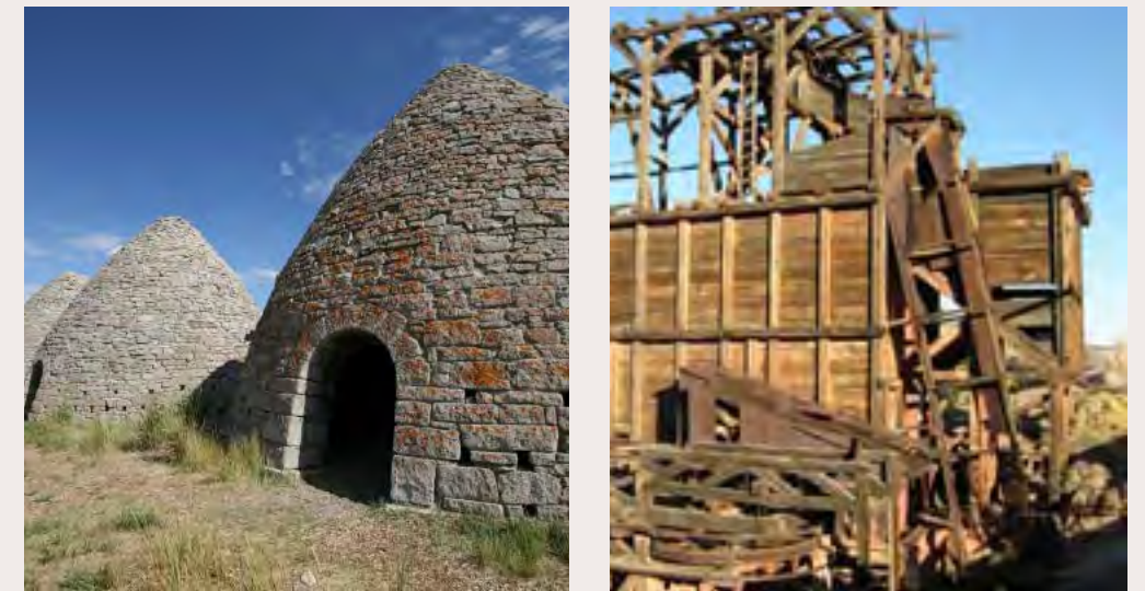
(1),(2) Colors and textures should be muted earth tones that echo hues of historic structures. Enhancements use cultural and geological elements as design inspiration.
