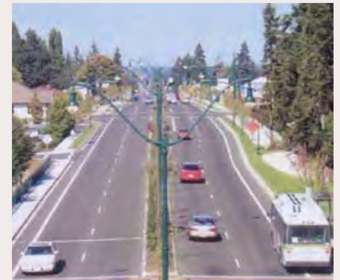
(3) After streetscape improvements.
