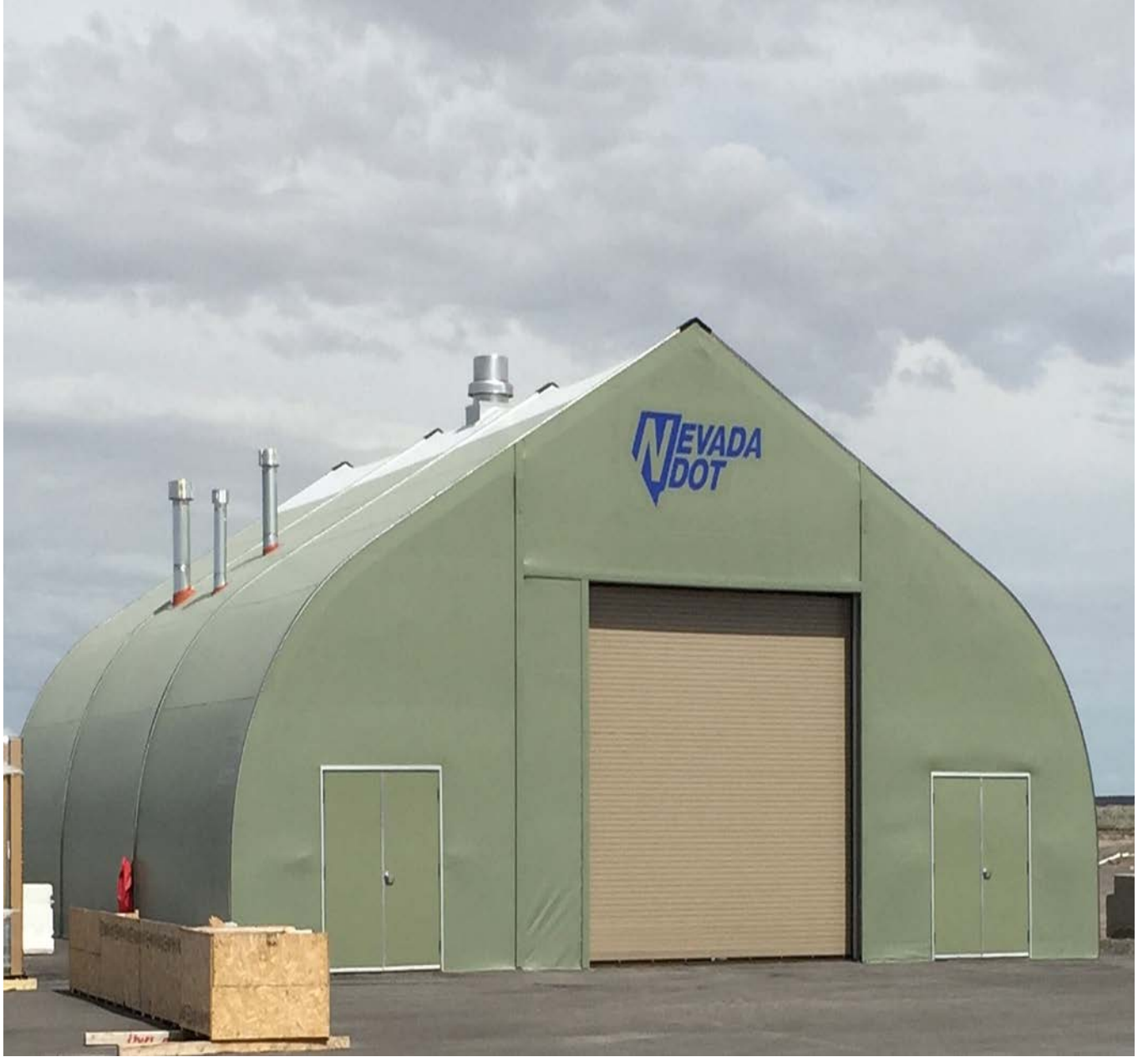
Self-contained equipment cleaning facility (Trento Yard)
