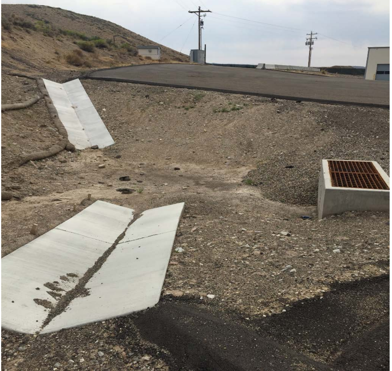
Stormwater sediment basin and various drainage improvements (North Fork Station)
