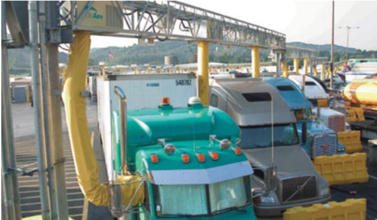
Figure 2.1 Truck Stop Electrification – Knoxville, TN
