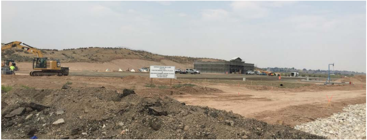
Figure 3.21 Golden Gate Travel Plaza Construction – Elko
