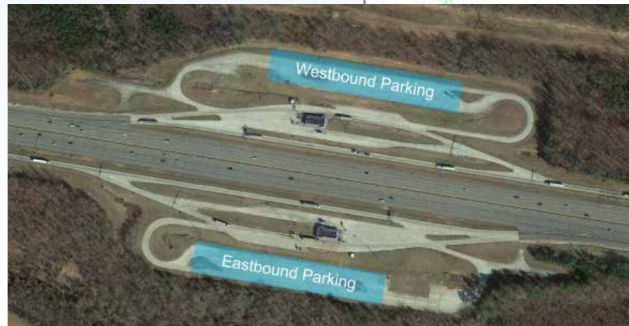
Parking at Weigh Stations I-40/I-85 (North Carolina) Source: CS
