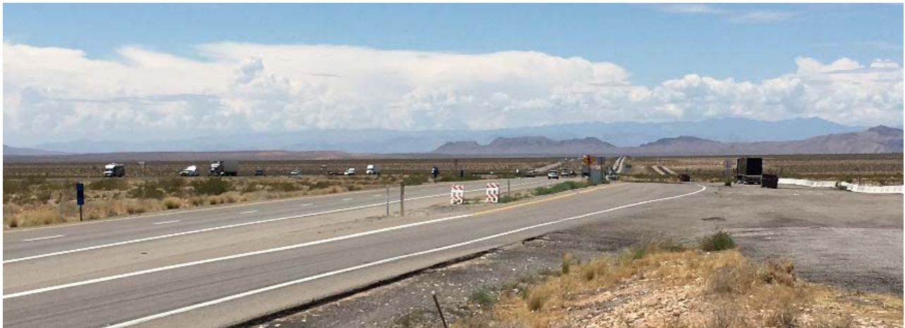
Figure 2.2 Authorized, Public, Unpaved, Unmarked Spaces at Truck Parking Pull-out (I-15, Top of Mormon Mesa)
