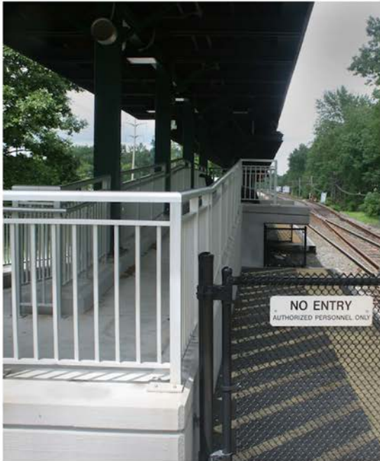
Mini-High Platform with Appropriate Barrier
