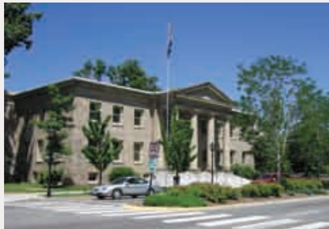
(2) The construction of the Carson City Freeway creates the opportunity to enhance streetscape amenities within the Historic Downtown/Capitol Mall area of Carson City. Wider sidewalks and pedestrian safety islands create a friendlier environment.
