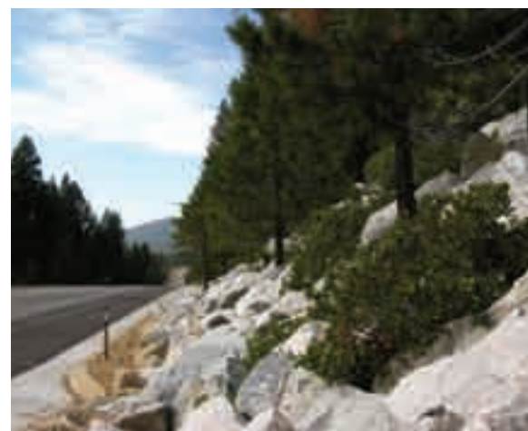
(3) Slopes should be treated with materials that match the context of surrounding landscape’s color and texture.
