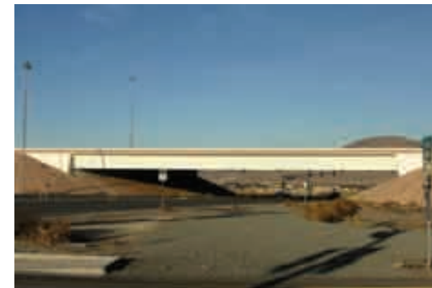
(4) The interchange with Mount Rose Highway (I-580/SR 431) establishes the entry into the Reno area. As the state's second largest metropolitan statistical area, highway structures should establish a sophisticated image.
