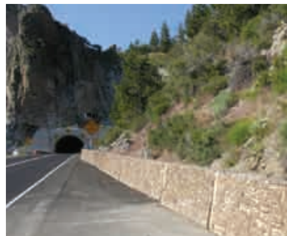
(7) Unique and scenic areas require that particular attention is given to the color and design of roadway structures to preserve the visual quality of the place.
