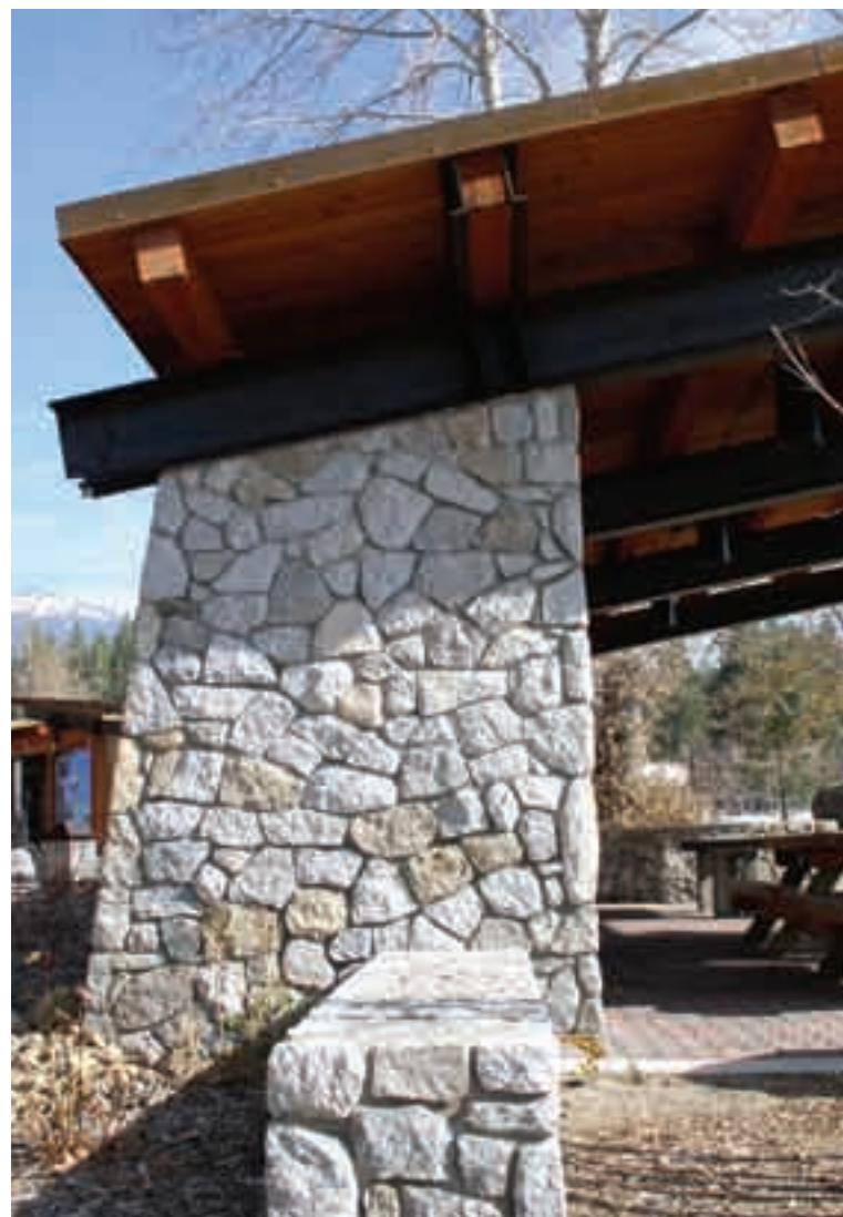
(6) Heavy stone foundations and exposed structural beams create structures that blend with the impressive scale of the surrounding landscape.
