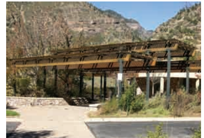
(2) Rest areas provide multiple opportunities for travelers. They serve many functions including, but not limited to, resting areas for travelers, viewpoints, trailheads, and staging area for recreationists.
