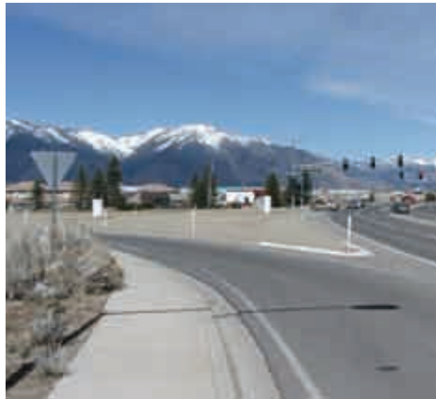
(1) The existing community entry into Minden lacks visual interest and is dominated by asphalt paving.
