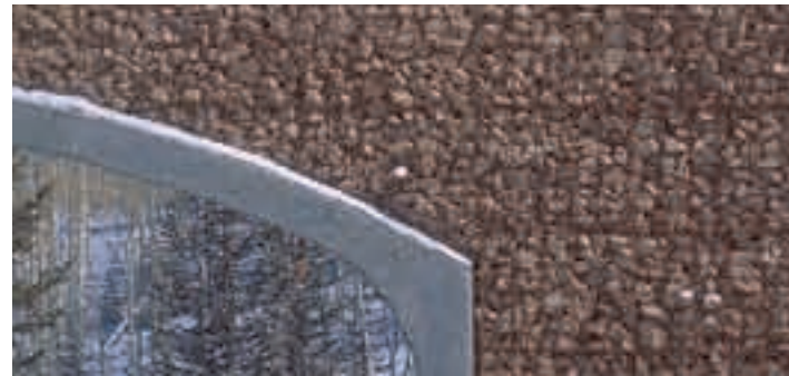
(4) Preferred gabion systems that utilize dark, muted stone. Wall should not appear to be an artificial system.
