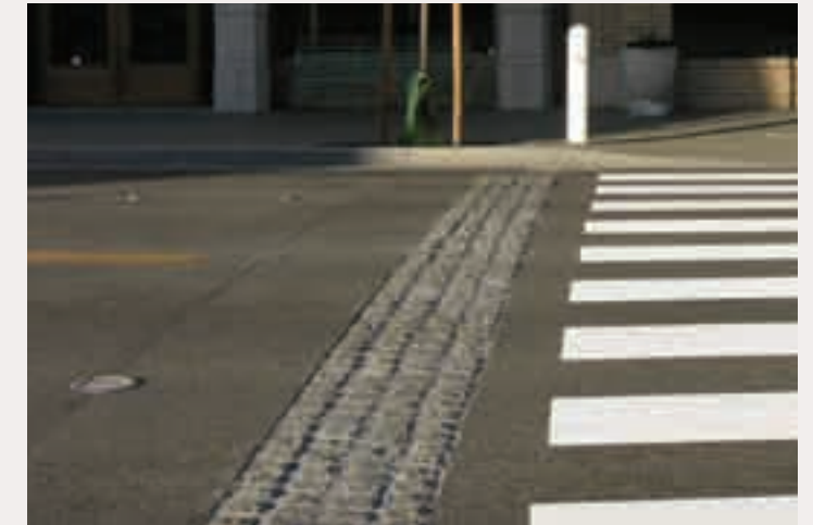
(2) Flashing pedestrian crossing signals enhance pedestrian visibility. In the image above, sensors on either side of the crosswalk activate flashing lights in the pavement when pedestrians cross the street.
