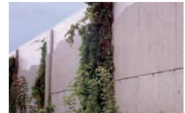
(7) The integration of vertical vegetation visually softens noise walls.
