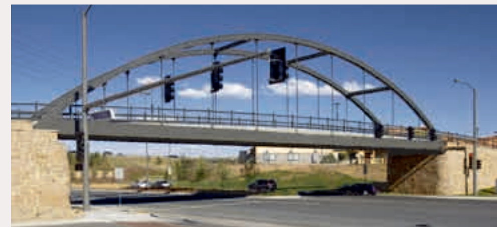
(11) Consider rail features and open bridge spans as part of bridge design to evoke a sense of character that relates to surrounding development and historical influences.
