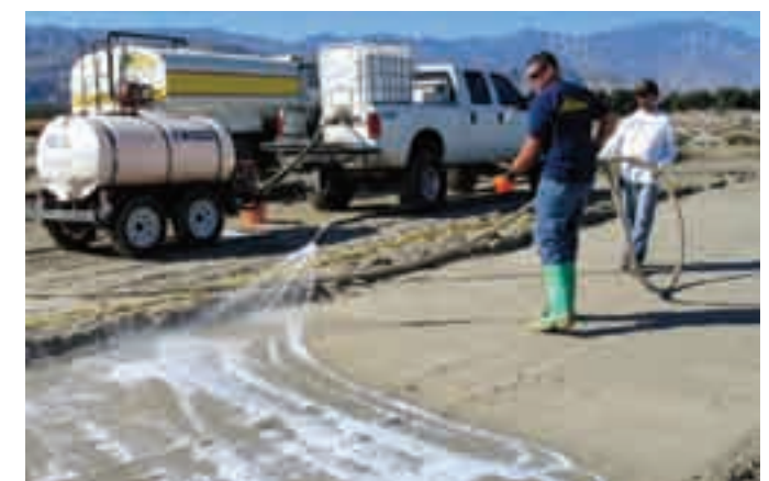
(2) Application of soil stabilizer aids in dust and erosion control.
