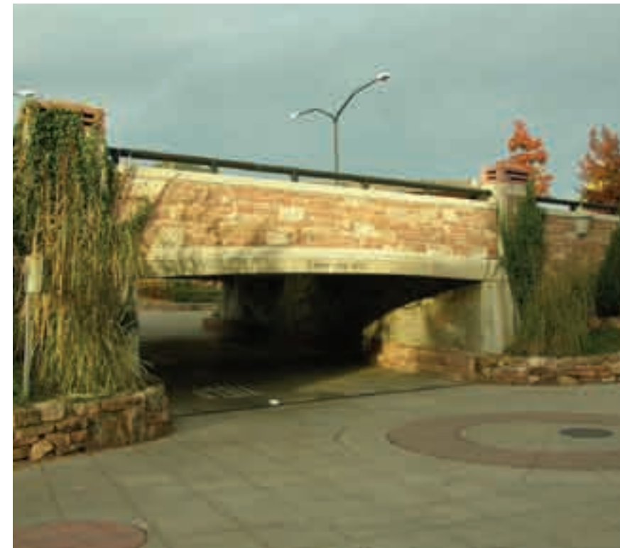
(1) The length of underpasses should be minimized where possible in order to allow natural lighting.
