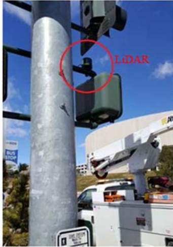
(a) Permanent installation (b) Temporary installation Figure 3-3 Different installation methods of roadside LiDAR sensors
