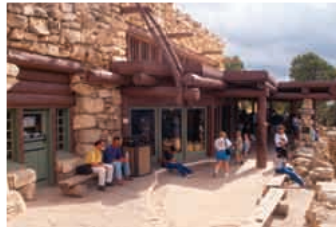
(2), (3) Road service facilities that use native desert materials and colors blend well into the existing desert landscape.
