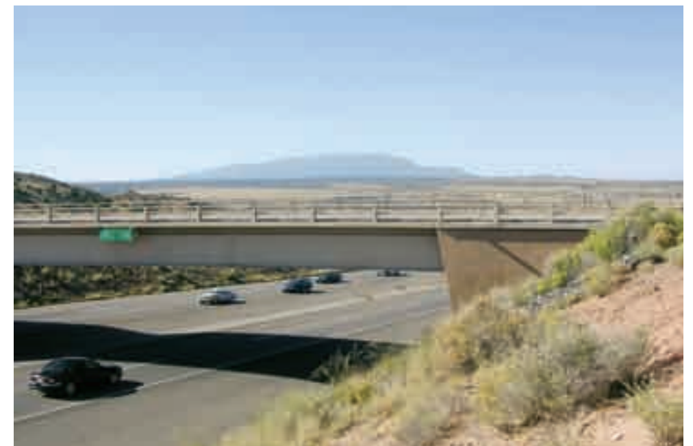
(6) Simple structural forms, earth-toned color palettes, and visually transparent rail designs help preserve the scenic character of the corridor.
