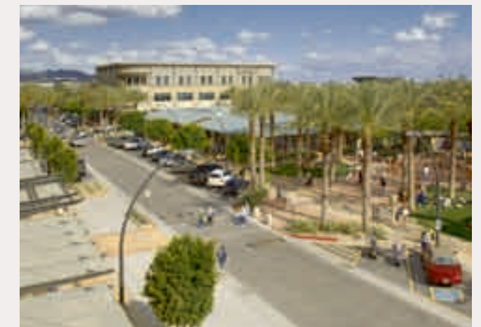
(2) Streetscape planting, varied paving materials, on-street parking, and enhanced lighting create a dynamic and vibrant community downtown experience.
