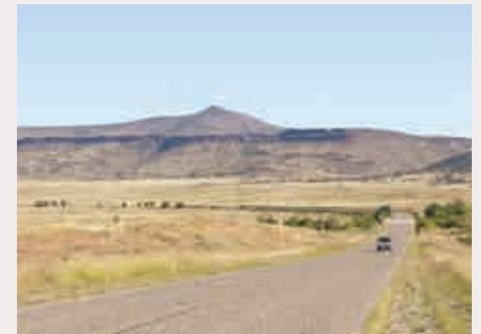
(1) Highway alignments can be designed to blend seamlessly into the existing topography and virtually disappear from view.
