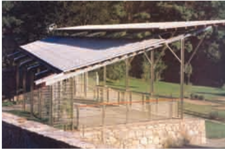
(1) Architecturally interesting shade structures and view platforms can attract more visitors and enhance their experience.
