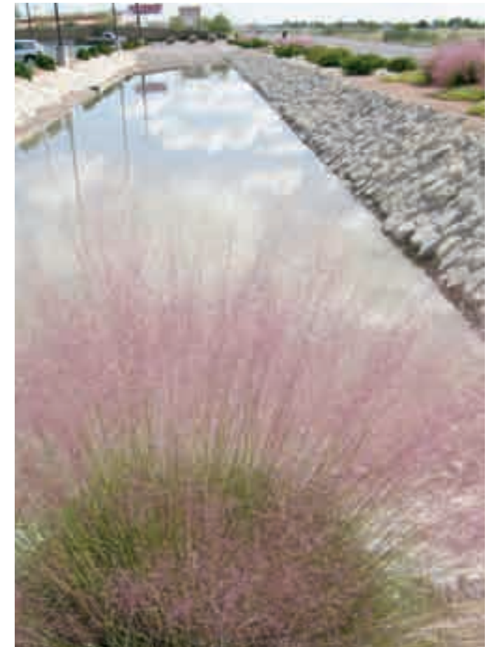
(7) Stormwater runoff can be harvested, stored, and reused to irrigate landscape plantings.
