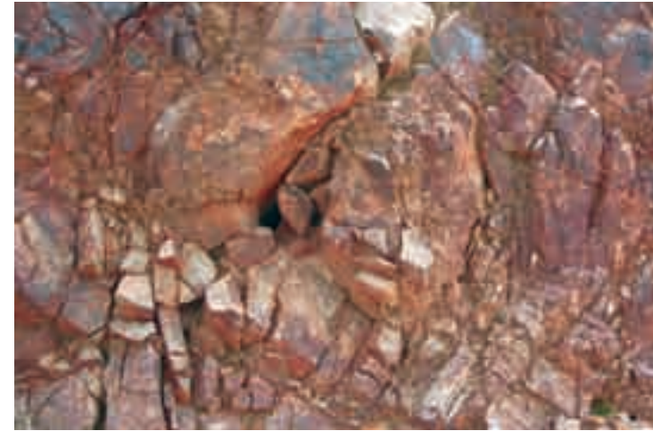
(3) Unnatural rock cuts should be stained to blend with the natural rock coloration.
