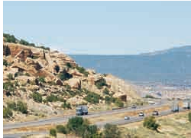
(2) Rock cuts and excavation should be designed to resemble natural rock formations in shape, form, and texture.
