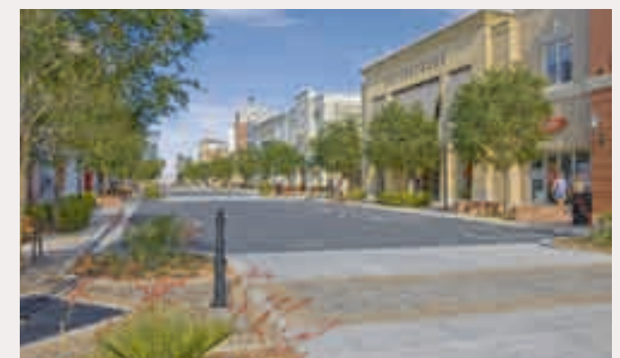
(6) Important road intersections and pedestrian crossings can be identified with stamped concrete or changes in paving material.
