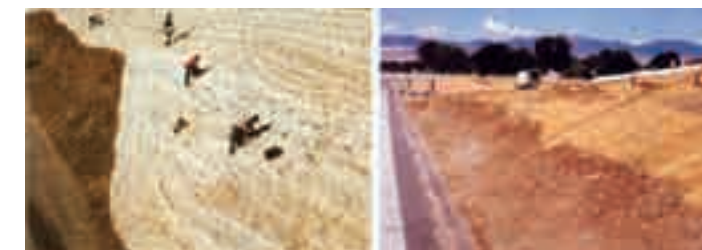
(1), (2) Application of geo-textile fabrics aid in erosion control.
