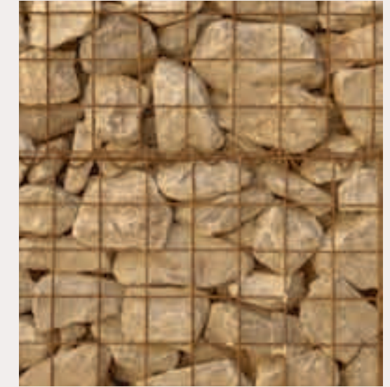
(3) When gabion walls are necessary, ensure that the wire and stone colors complement one another and the surrounding landscape.
