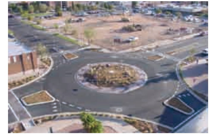
(3) Pedestrian crossings at roundabouts require additional identification through striping and paving changes due to the unique geometry of these intersections.
