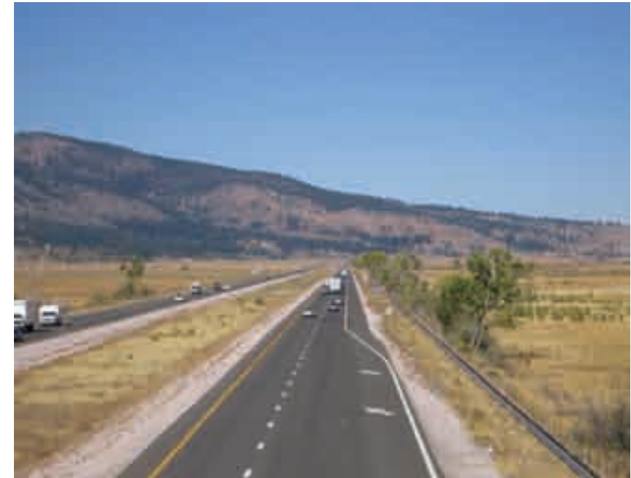
(1) Native revegetation is appropriate for highway medians in rural settings.
