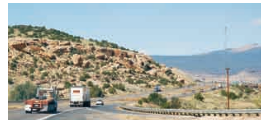
(2) Re-sculpted rock cuts change artificial slope banks into naturally occurring landforms. Plan cuts that terrace, bench, and use bedding planes found in existing rock formations.
