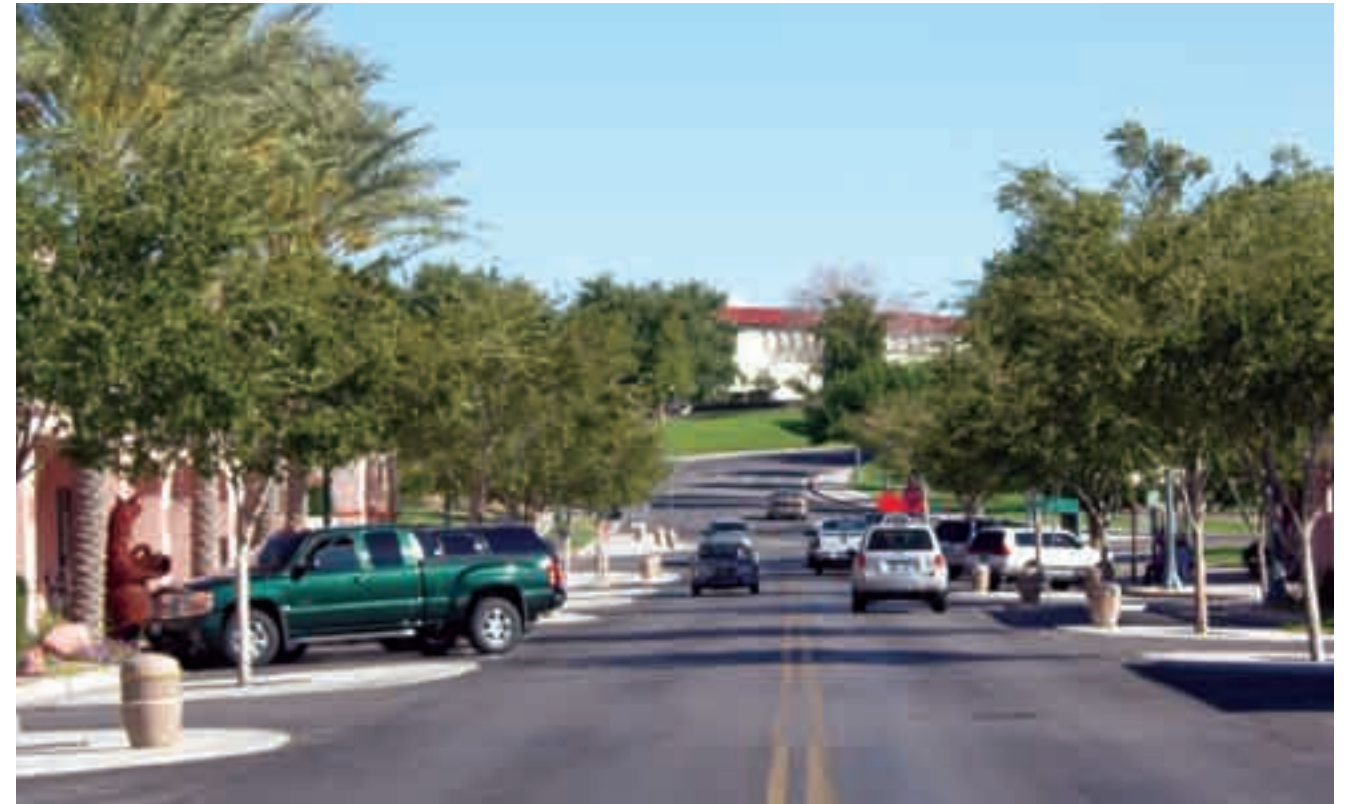
(1) Street elements such as on-street parking, bollards, landscaping, and bulb-outs delineate distinct zones for automobiles and pedestrians and provide visual cues to slow down.
