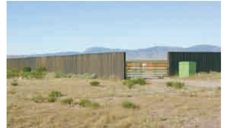
(1) Screening maintenance facilities from the road is recommended and helps minimize visual clutter in the traveler's view of the larger landscape.
