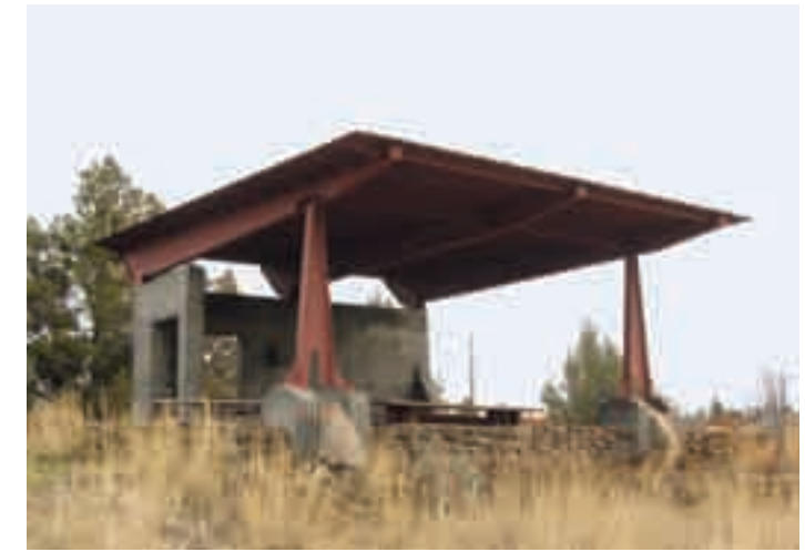
(3) Self-weathering materials should be used for architectural elements at rest areas and viewpoints.
