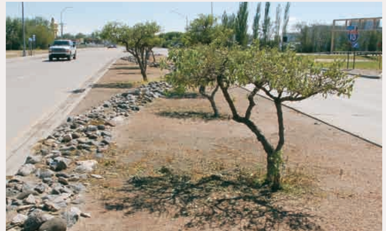
(1), (2) Medians should be designed to accommodate stormwater runoff where possible and be planted with low maintenance, drought-resistant plant materials.
