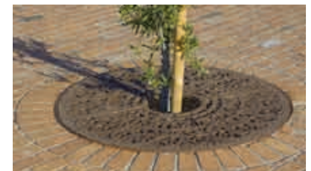
(4) Tree grates protect trees from unwanted root compaction along street environments.
