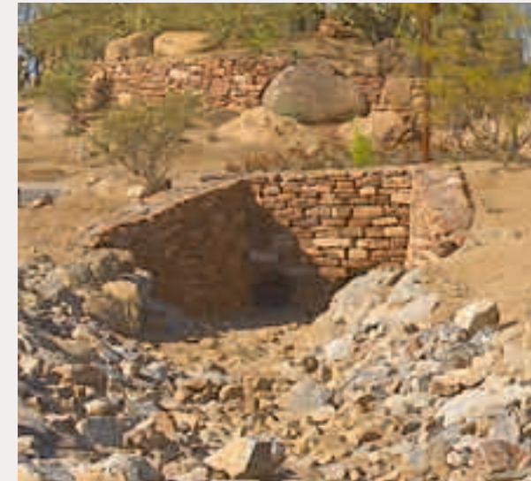
(1), (2) Rock bed drainage reduces erosion, allows some water to infiltrate, and can provide irrigation for adjacent plant materials.
