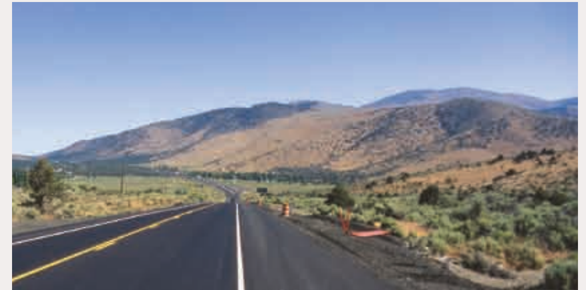
(1) The placement of asphalt millings on the highway shoulder creates a stark contrast between the road and the adjacent undisturbed landscape and should be avoided.
