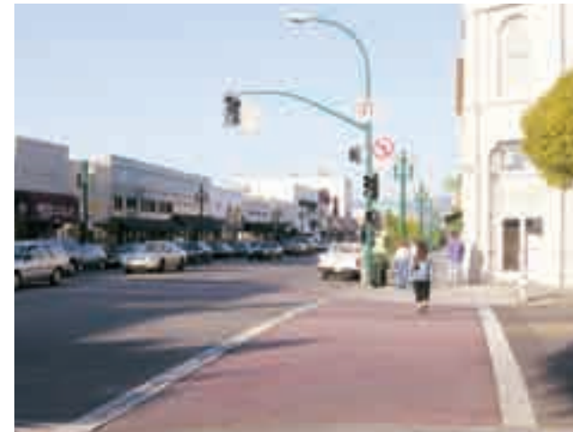
(3) Contrasts in paving color and texture indicate to motorists that they are approaching a pedestrian crossing.
