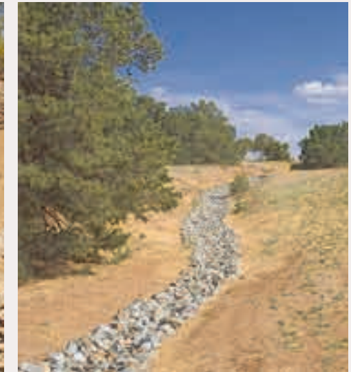
(1), (2) Rock bed drainage reduces erosion, allows some water to infiltrate, and can provide irrigation for adjacent plant materials.
