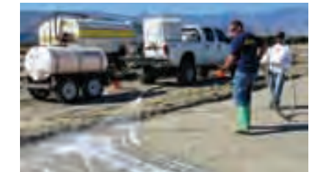
(3) Application of soil stabilizer aids in dust and erosion control.
