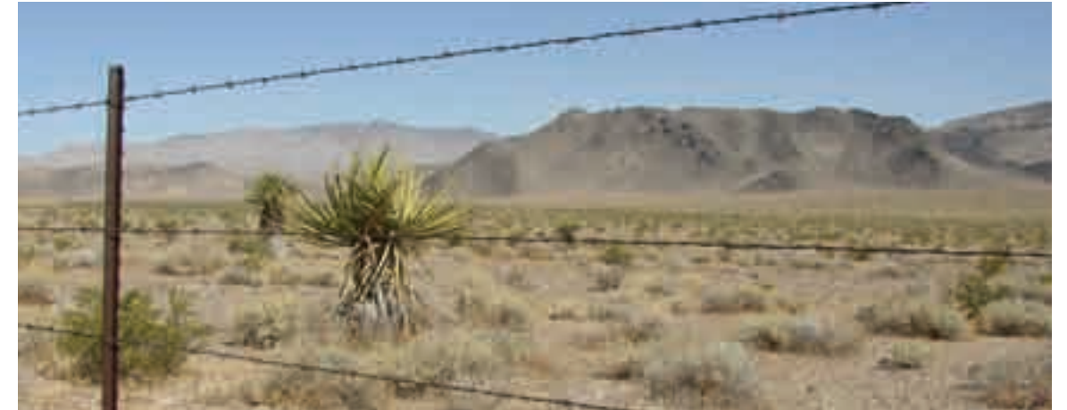
(1) Three-strand fencing maintains the rustic character of the rural segments of the corridor and minimizes the visual impact of fencing on the driver.
