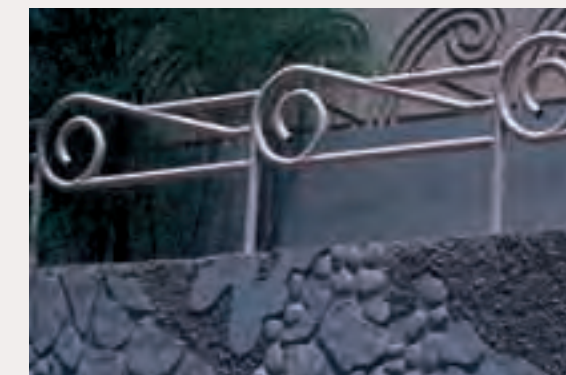
(4) Form-lined concrete and decorative railings can be used to create a desert visual design theme.
