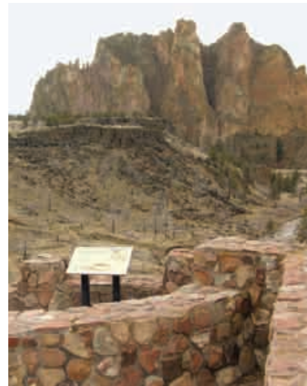
(2) Viewpoints should be placed at key viewing areas, and built with materials and forms reflective of their surroundings.
