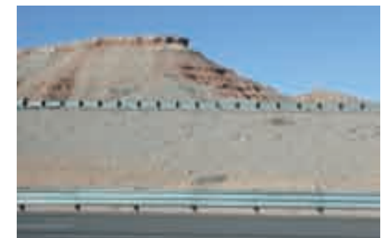
(1) Acid-washed steel guardrail blends into the surrounding landscape better than shiny galvanized steel.
