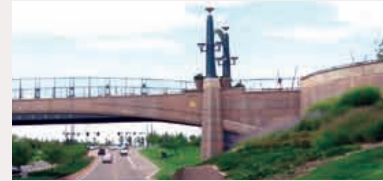
(1) Lights can be incorporated in the bridge design as a feature of the approach.
