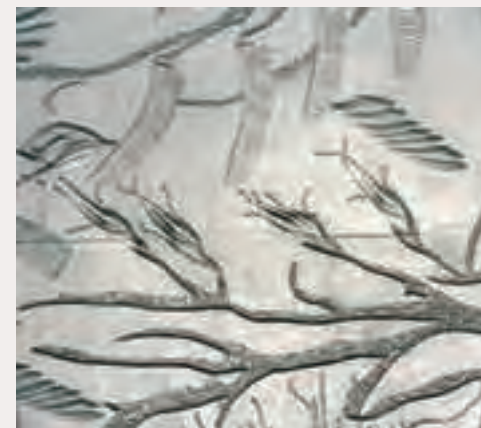
(3) Form liners can be used to produce details in wall patterns.
