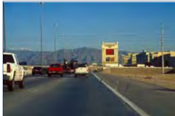
(1) This is an example of existing conditions along I-15 approaching the resort corridor. A lack of planting and earthwork exposes several visually disruptive elements such as power lines and light poles.
