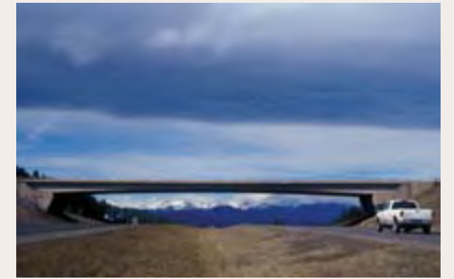
(1) This bridge on I-70 near the continental divide in Colorado was constructed without center piers to frame the view of the mountain range beyond. This underpass window enhances the view for the driver.
