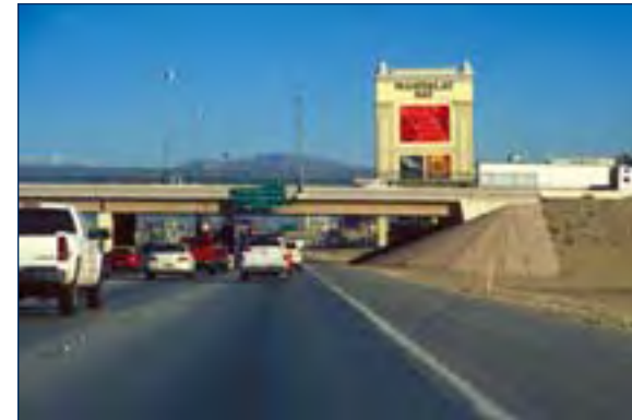
(3) High mast lighting, slope paving, and inconsistent materials currently detract from the visual quality of the resort district.
