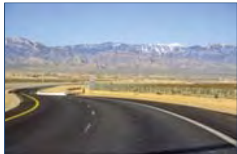
(1) This is an example of existing conditions at I-215.
