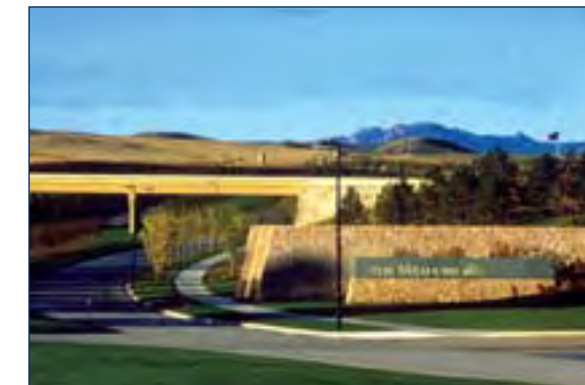
(4) Example of a community gateway incorporated into retaining wall and bridge structure.
