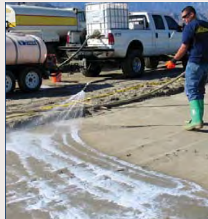
(5) Application of soil stabilizer aids in dust and erosion control.
