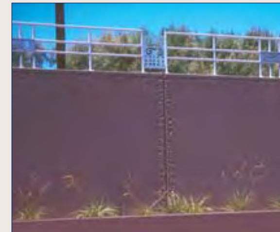
(5) Simple retaining wall patterning, railing design, and landscape palette. The wall is separated from the concrete barrier by a space and planting area.
