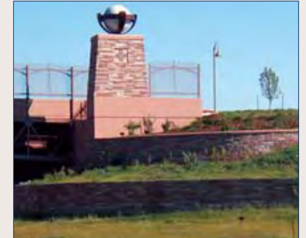
(3) Bridge design integrated into retaining wall with landscape planting to create moderately steep slopes and terraces for planting.
