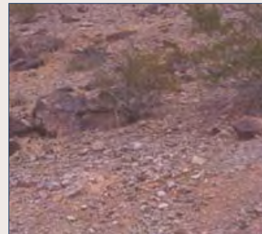
(3), (4) A mix of aggregate size and color re-establishes the graded slope to a naturalized condition.
