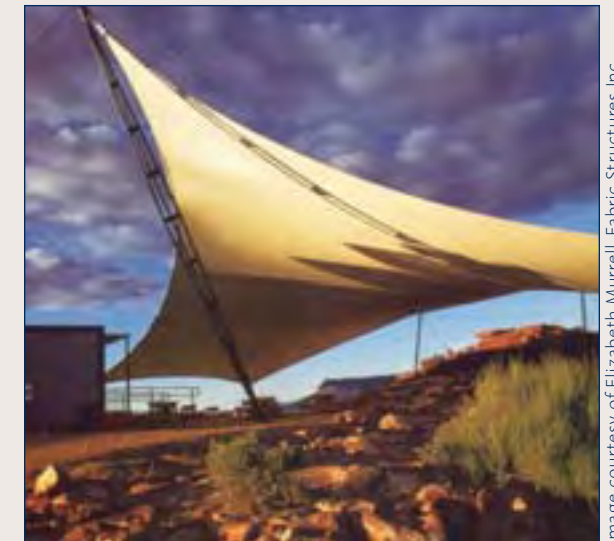
(2) Notable outdoor space and welcome center entry feature example.
