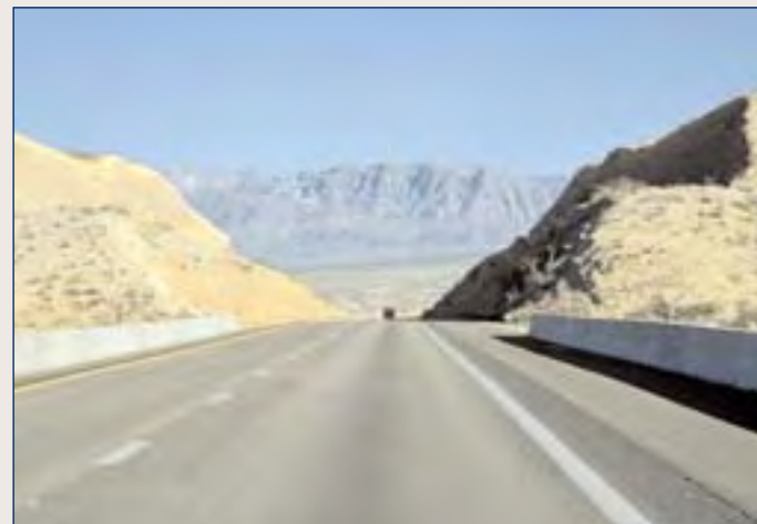
(3) Artificial terracing in an existing road cut creates poor visual appearance.
