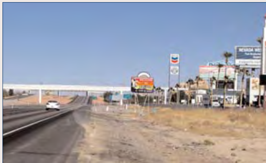
(5) Existing conditions at Nevada stateline.
