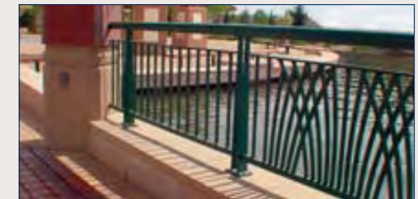
(7) Custom pedestrian bridge rail highlights crossing point.
