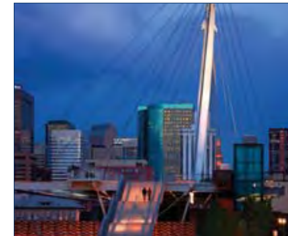
(2) This unique pedestrian overpass provides an example of a bridge feature that is used to create a "landmark" for a community gateway.
