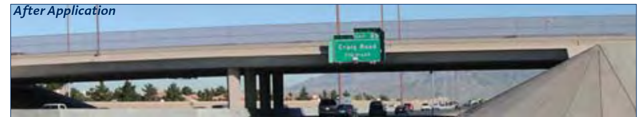
(1), (2) Appropriate coloring of bridge enhances visually quality
