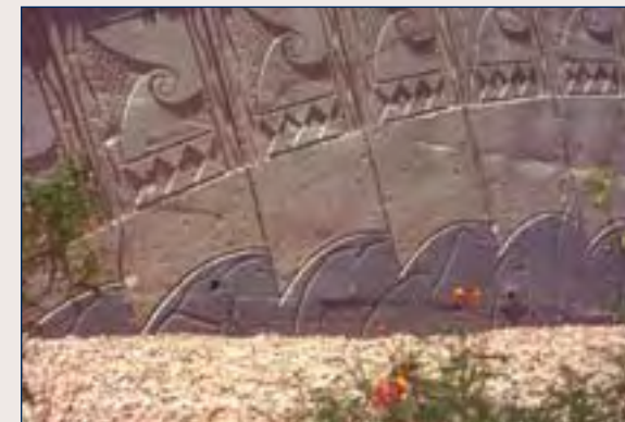
(3) Sound wall with decorative imprint motif created with custom form liner. This is both imprint as well as "additive relief" to project beyond the wall surface.
