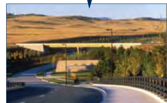
(1), (2), (3), (4) This series of highway design studies shows the process of visualization from computer modeling to the built project.
