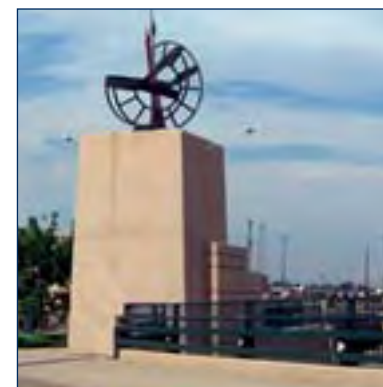
(6) This is an example of a landmark bridge detail.
