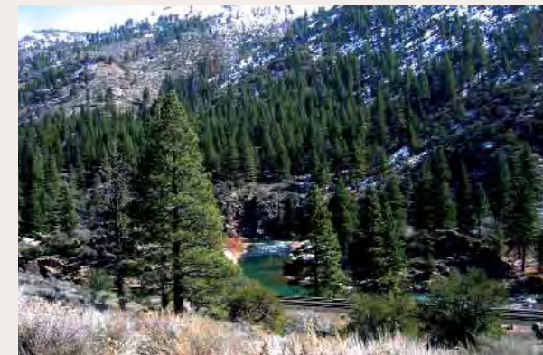
(1) Extending from the California/Nevada border to Mogul, the Sierra Nevada Passage Design Segment provides a dramatic entry into the Reno/Sparks urbanized area.
