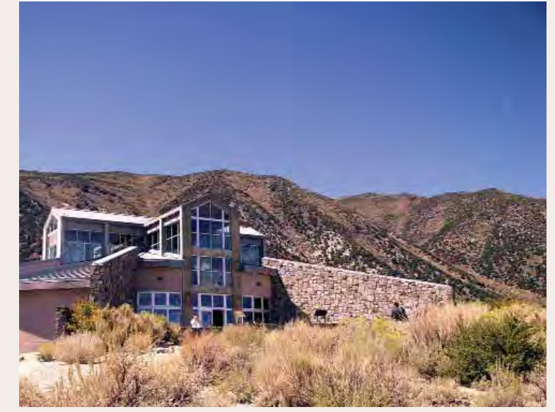
(5) The statewide welcome center should subtly blend into the surrounding landscape in order to capitalize on the natural beauty of the corridor.
