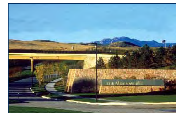
(5) Example of a community gateway incorporated into retaining wall and bridge structure.
