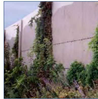
(2) The integration of vertical vegetation softens sound walls.
