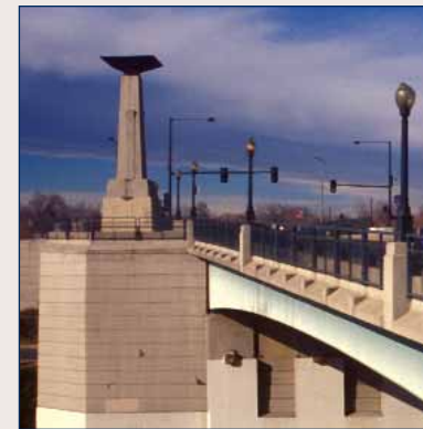
(6) Landmark bridge detail in urban areas.
