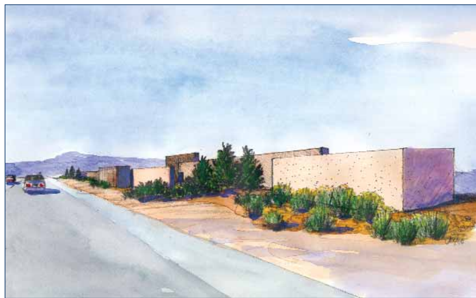
(3) This sequence of travel over approximately 1000 feet illustrates the sound wall design for the corridor. Characteristics include staggered wall planes, landscape planting in front of the wall face, and patterning on the wall face.
