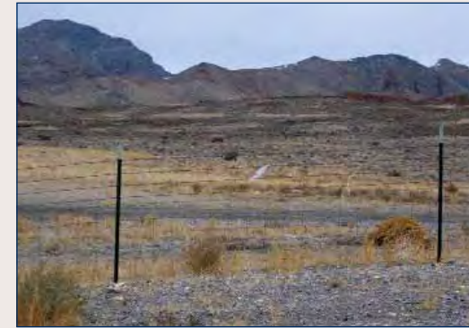
(1) Three-strand fencing should be used within the rural segments of the corridor.
