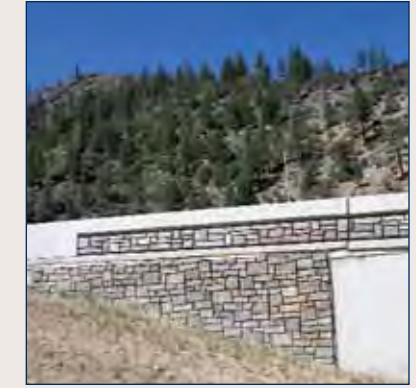
(5) Bridge features reflect local stone materials.
