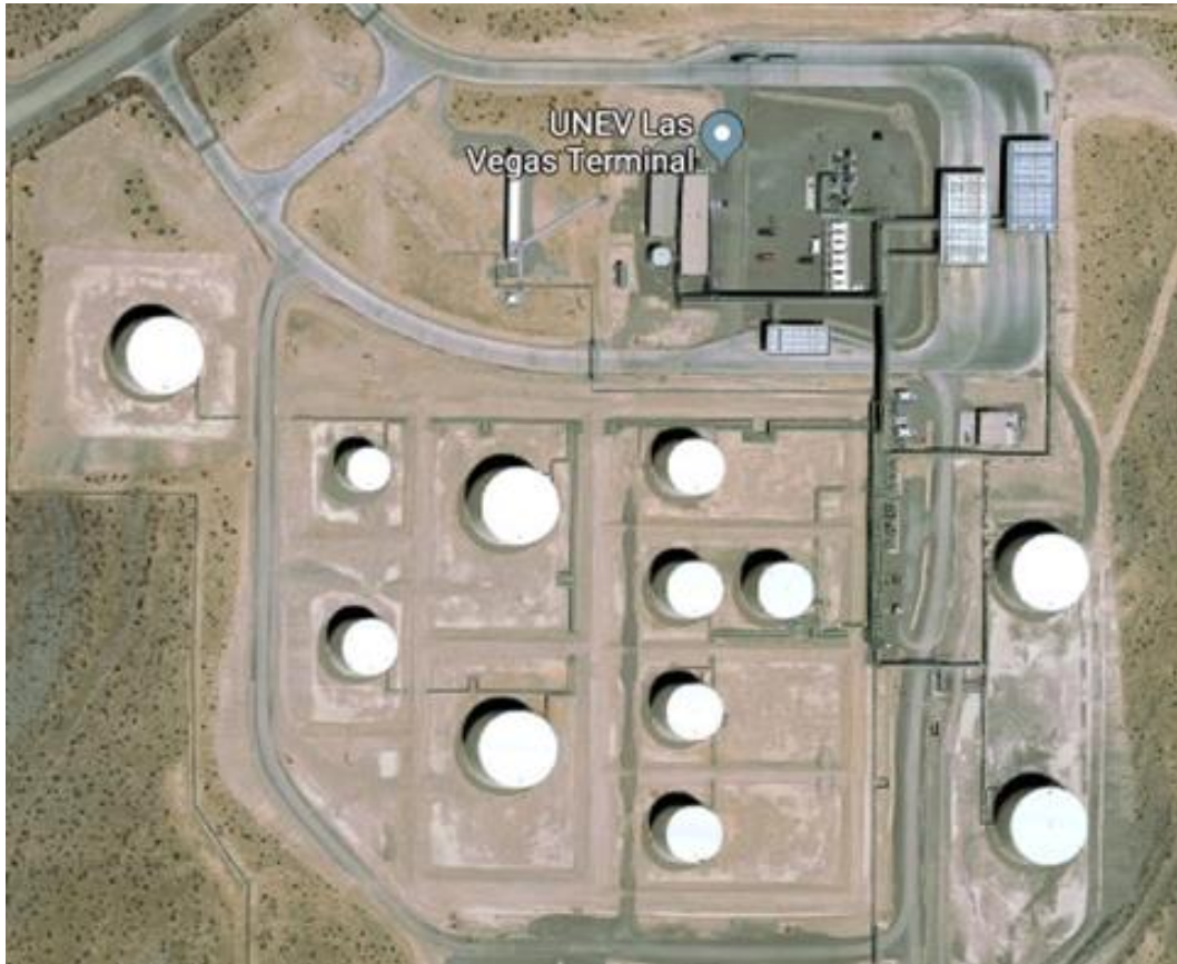
Figure 3.3 Holly Energy Terminal, Apex Industrial Park
