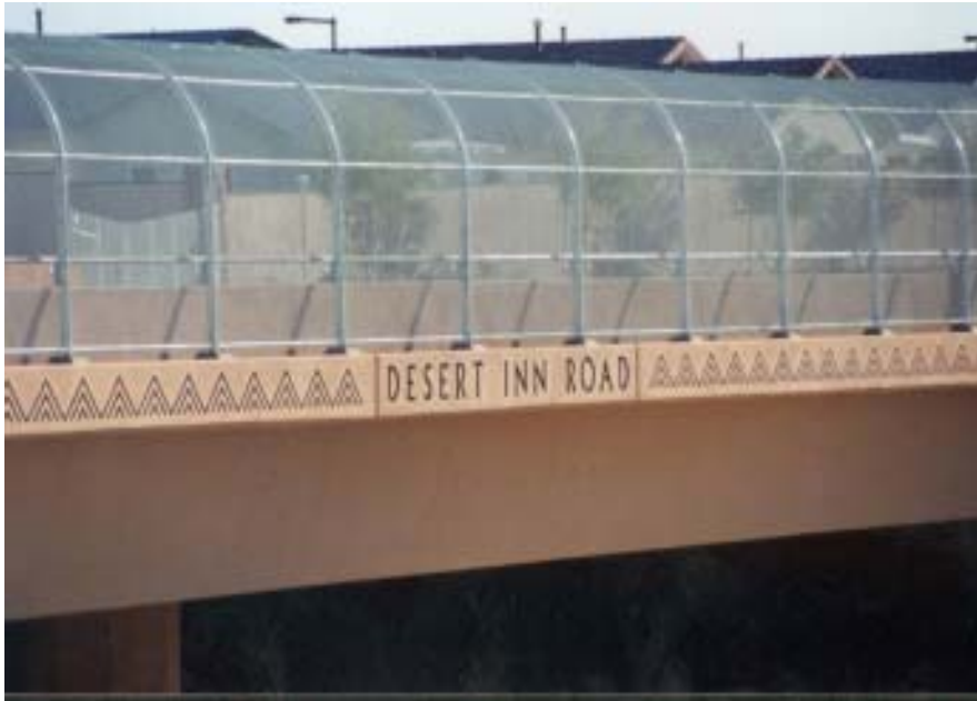
Desert Inn Road overpass on the Clark County Beltway.
