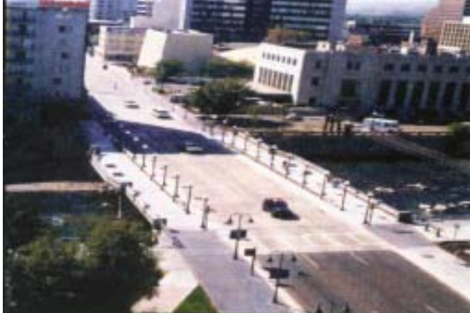
Center Street Bridge, Reno.
