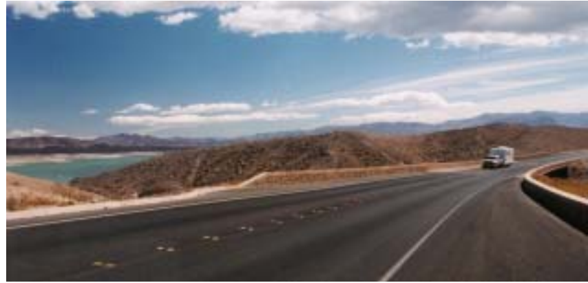
SR 166, Lakeshore Road, Lake Mead National Recreation Area Pre-cast concrete barrier respects the 1930's heritage of Lake Mead, meets current safety standards, and blends into the landscape (detail below).
