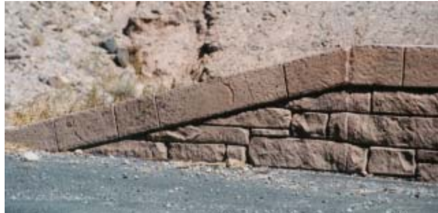
SR 166, Lakeshore Road, Lake Mead National Recreation Area Pre-cast concrete barrier respects the 1930's heritage of Lake Mead, meets current safety standards, and blends into the landscape (detail below).
