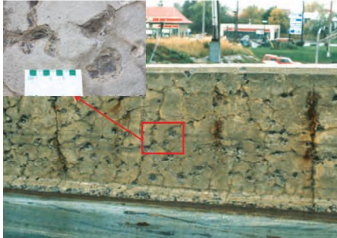
Figure 1.9: Map-cracking along with several pop-outs caused by particles of shaly limestone (from Thomas et al., 2013)
