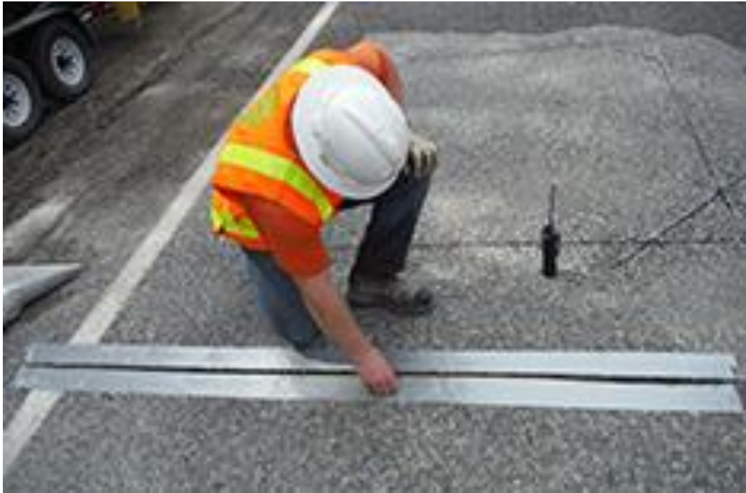
Figure 4.1 Installing In-Pavement Traffic Counter
