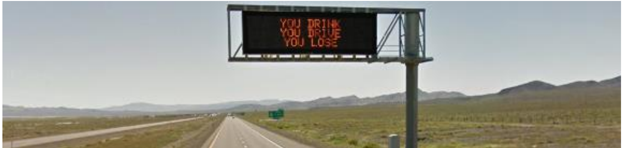
Figure 5.1 Dynamic Message Sign (I-80 westbound) Near Exit 83 (Fallon)
