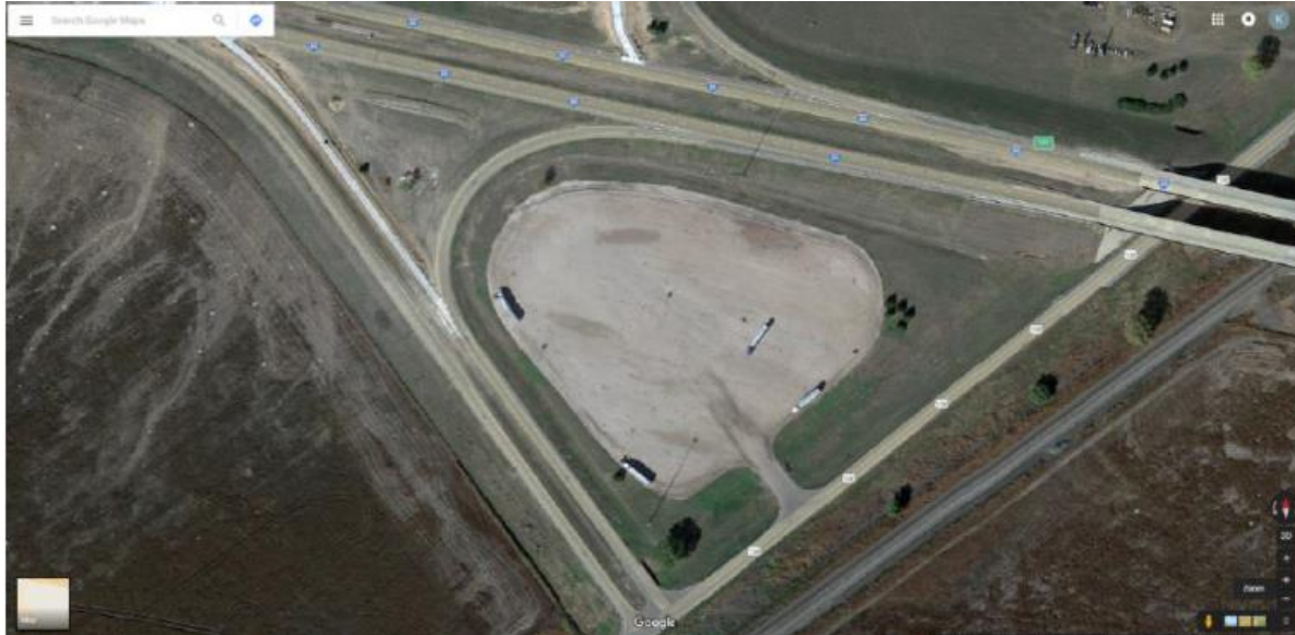
Figure 2.5 Truck Parking Inside Interchange Half Cloverleaf I-80, Big Springs, NE
