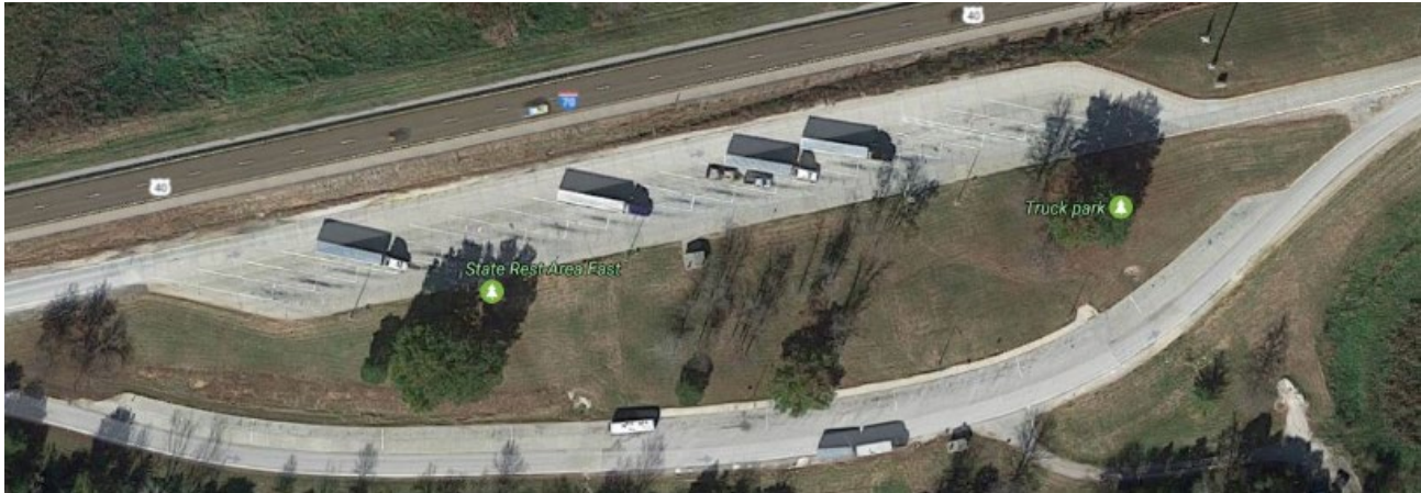
Figure 2.7 Missouri Converted Rest Area I-70
