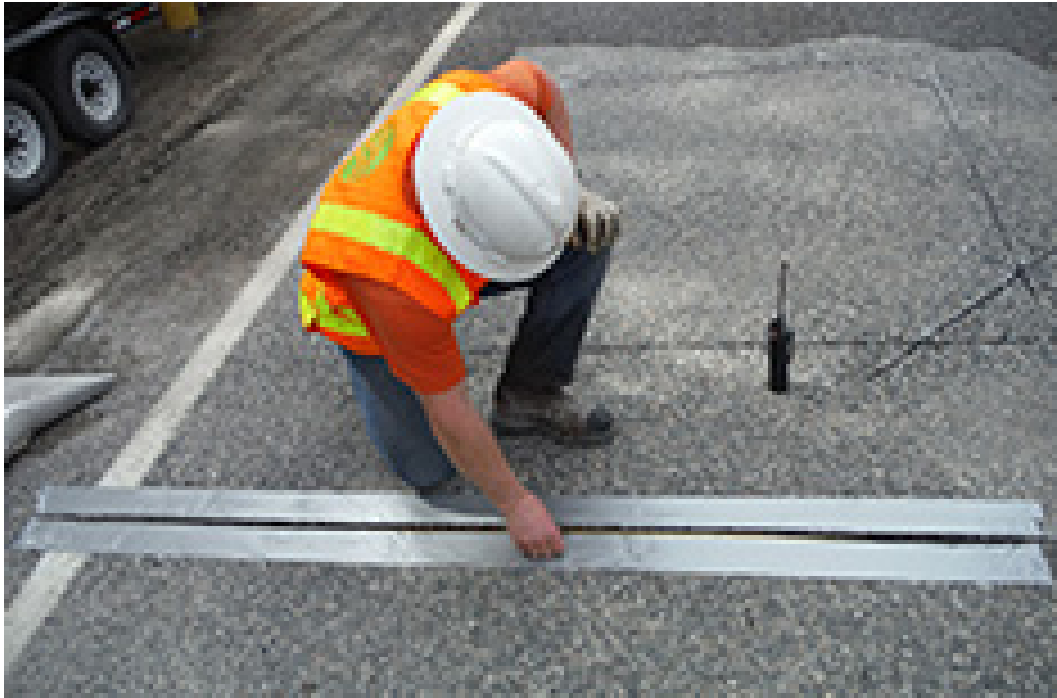
Figure 4.1 Installing In-Pavement Traffic Counter
