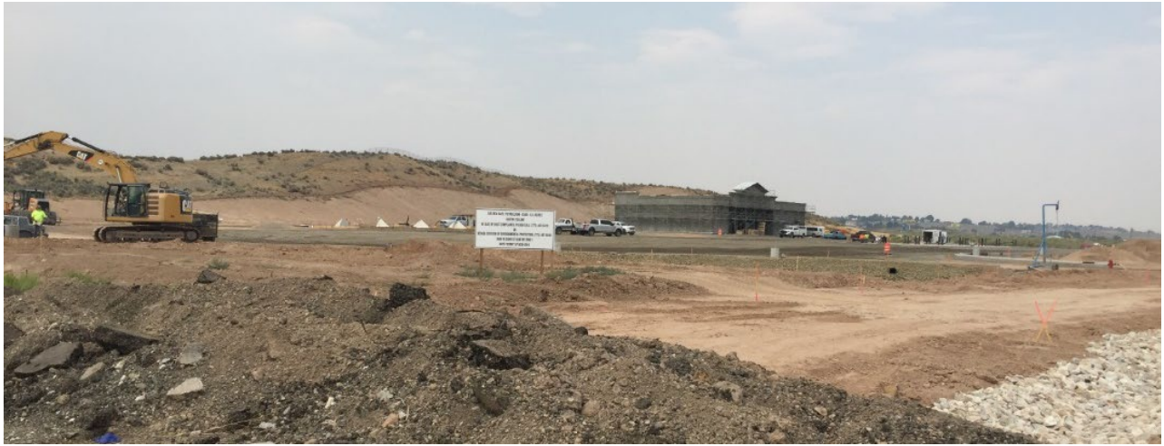
Figure 3.21 Golden Gate Travel Plaza Construction – Elko
