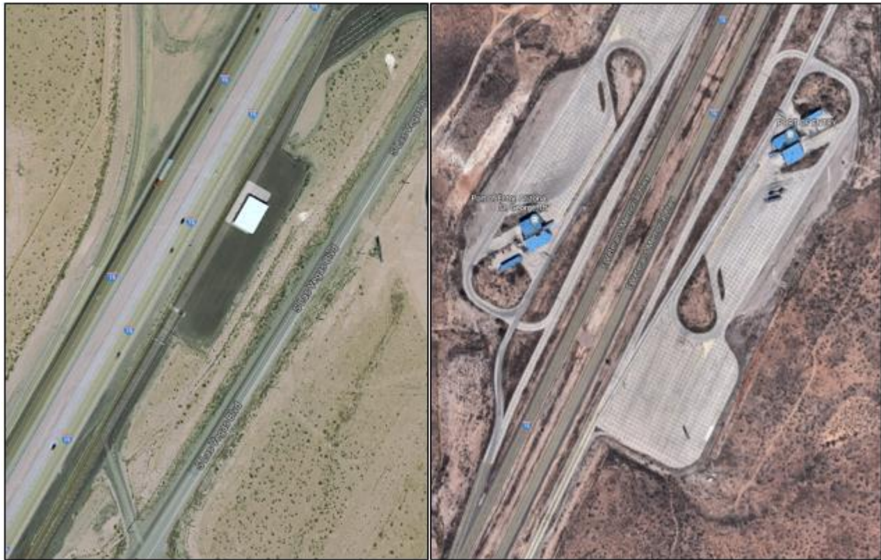
Figure 2.6 Sloan Inspection Site, NV (Left) and St. George Port of Entry, UT (Right)
