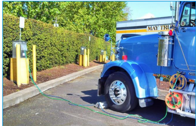
Truck Stop Electrification
