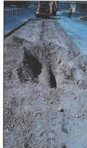
Maintenance activity to repair a section of deteriorated storm drain on Great Basin Boulevard
