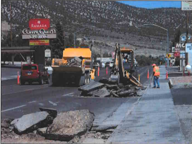
Maintenance activity to repair a section of deteriorated storm drain on Great Basin Boulevard
