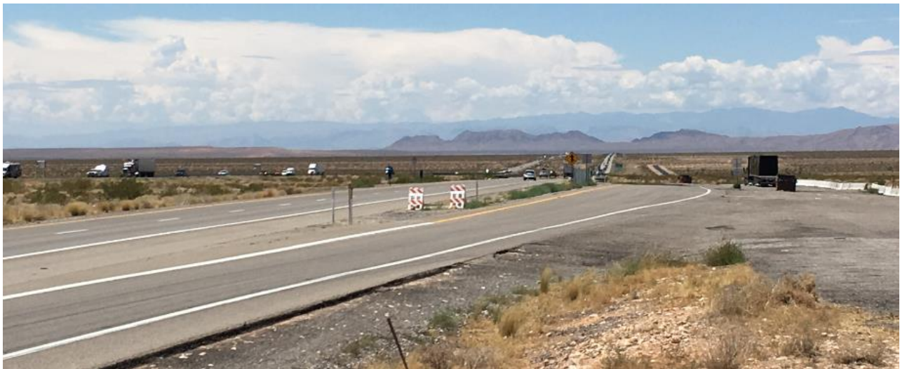
Figure 7.1 Mile Marker 110 (Mormon Mesa) Truck Pull-Off/Turnout I-15 Southbound
