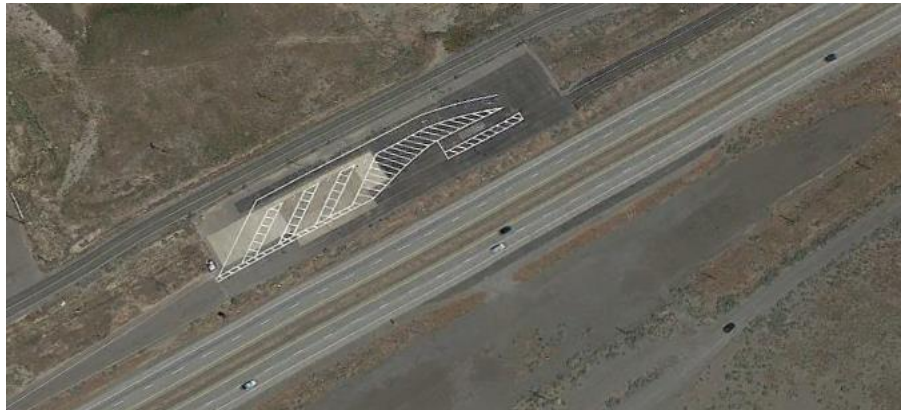
Mustang Inspection Site 0151—NHP facility that is no longer in use. Recommended for conversion to truck parking. I-80 westbound, Washoe County.
