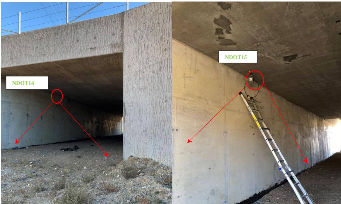
Figure 2-6 Locations and directions of the cameras at the north Wildlife Underpass on USA Parkway
