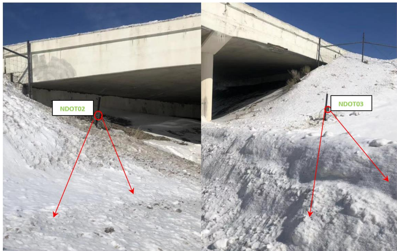
Figure 2-8 Locations and directions of two cameras at the west vehicle underpass in the Pequop Mountain (2019 spring)
