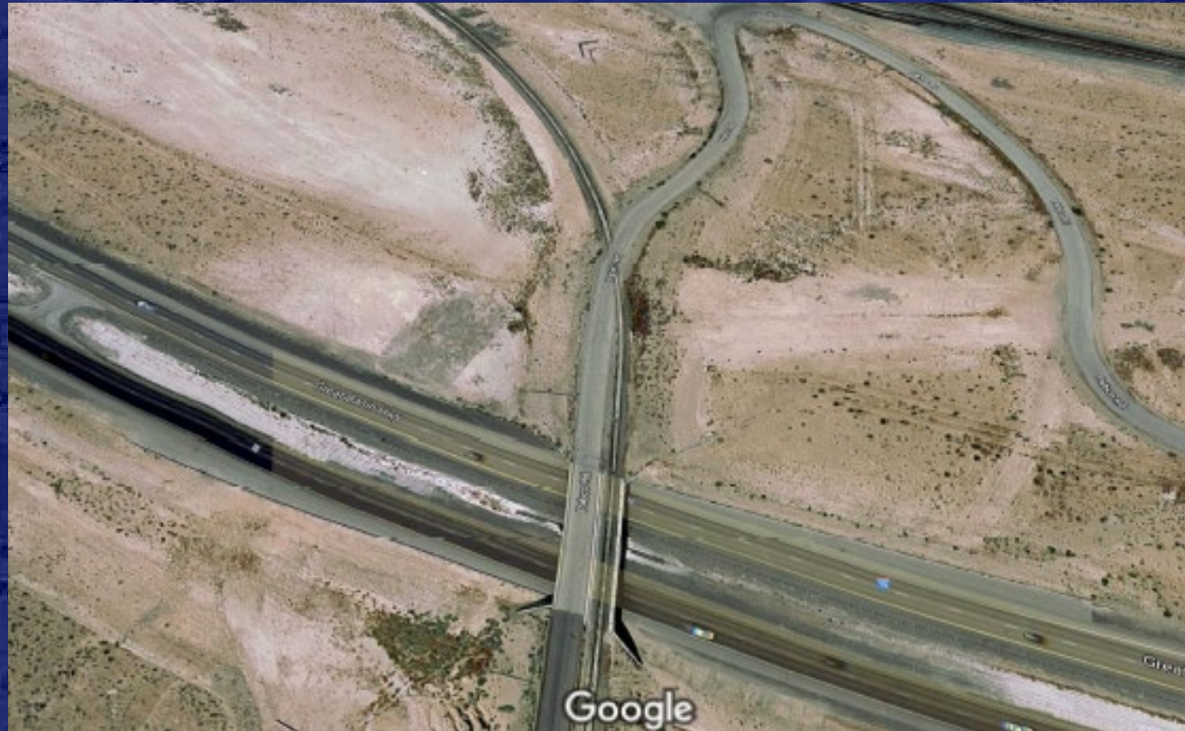
Looking down on Pabco Road (H-970 Apex Grade Separation, MP 60.31) and UPRR (G-1041 Apex UPRR Spur UP, MP 60.32)
