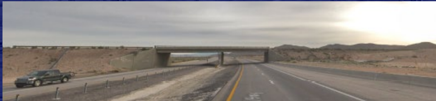
Looking Northeast on I-15 at Pabco Road Grade Separation, MP 60.31
