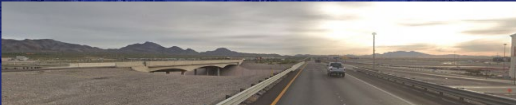
Looking Northeast on I-15 at Speedway-I-965N/S Speedway BI, MP 53.64
