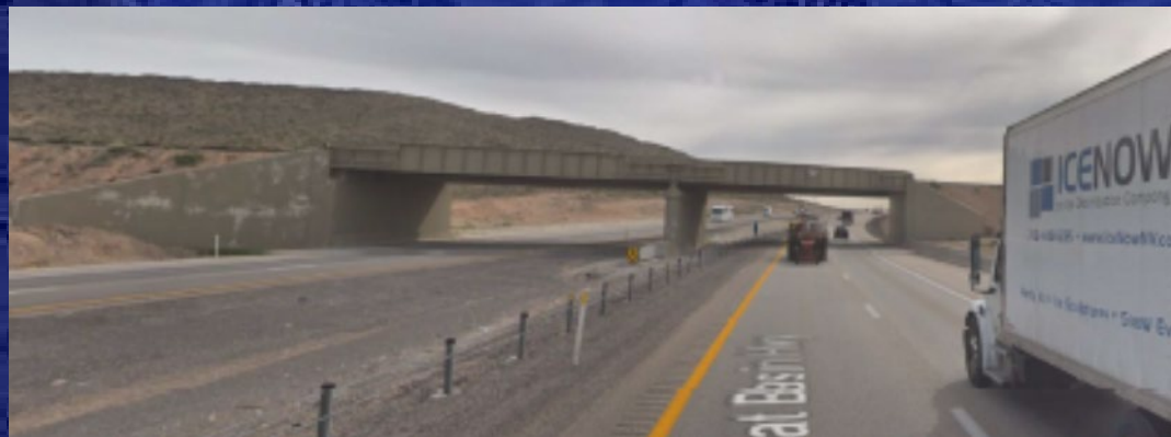
Looking Southwest on I-15 at G-1041 Apex UPRR Spur, MP 60.32
