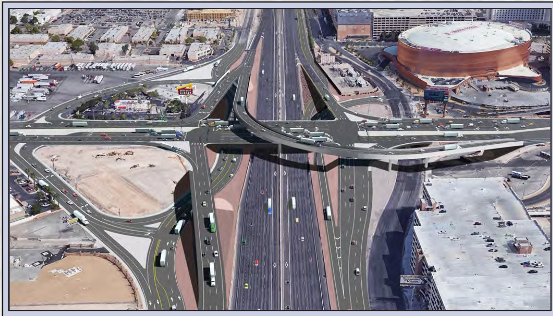
View looking north of the Tropicana Interchange improvements..
