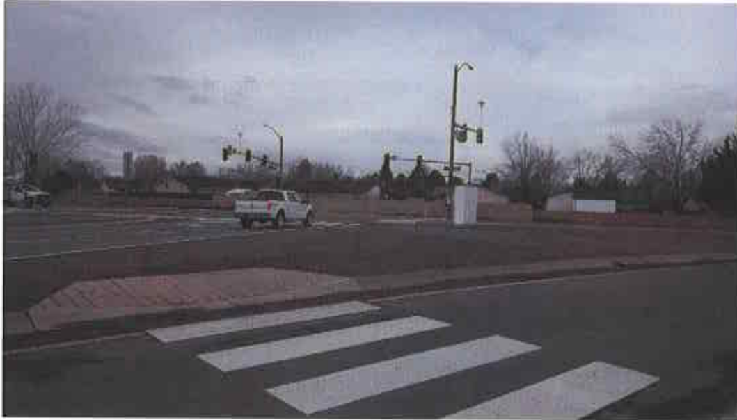
Figure 2. The intersection presents several traffic medians, traffic lights and light poles (approximately 60 feet in height), and pedestrian crossings. View west.
