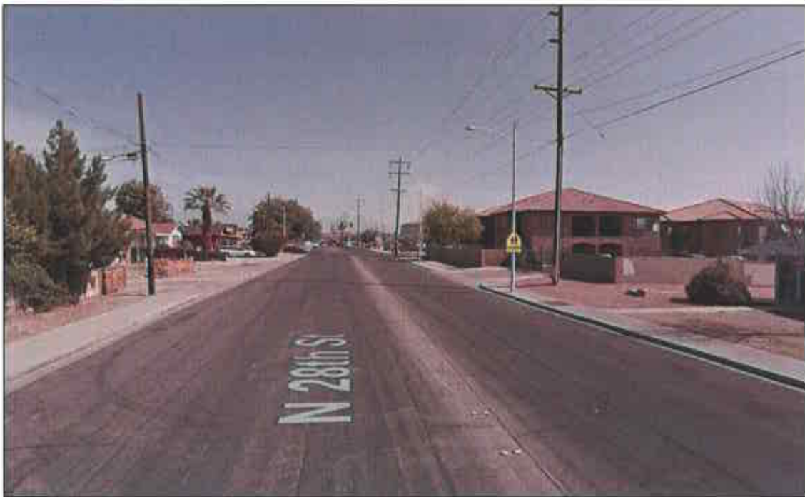
Figure 2. 28th Street just north of Valley Street, looking north.
