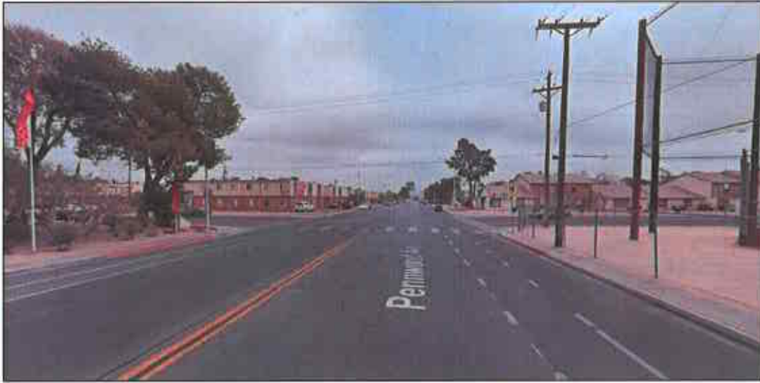
Figure 3. Pennwood Avenue and Wing Street intersection, looking east.
