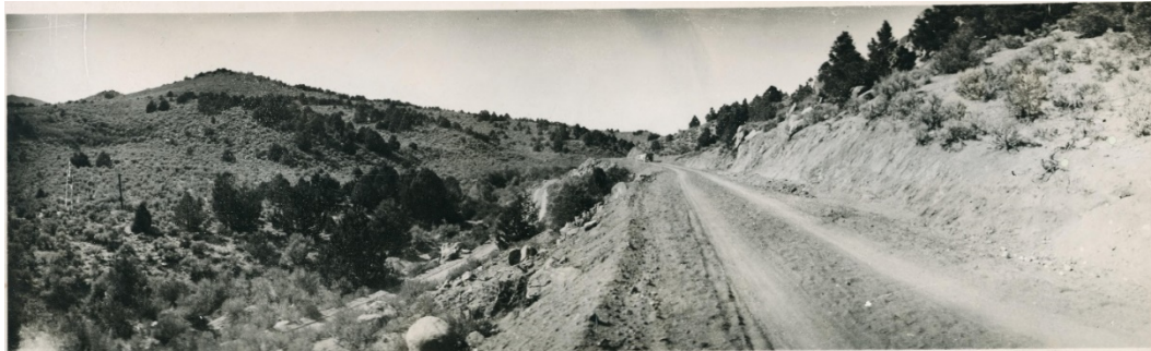
Figure 14. Toiyabe Forest Road showing old (at left) and new (at right) alignments, 1920. 118
