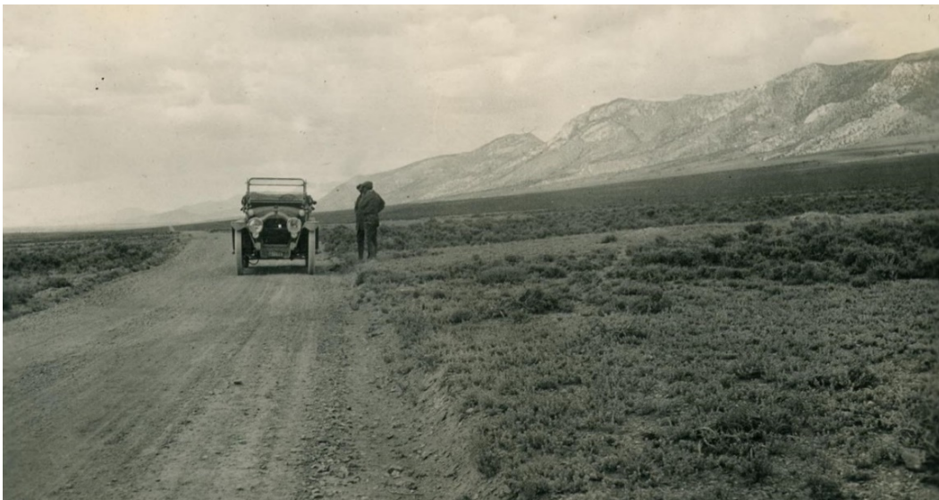
Figure 5. The Lincoln Highway east of Ely illustrating unimproved earth roadbed, 1915. 57
