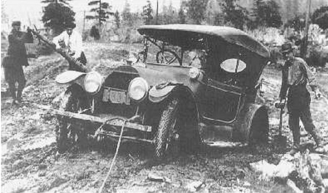
Figure 2. Image illustrating poor condition of many early-twentieth-century roads. 12
