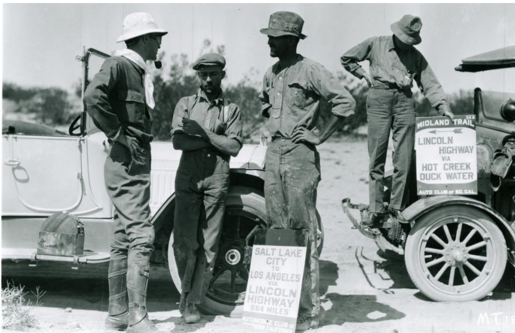
Figure 6. Crew of the Automobile Club of Southern California placing signs on the Midland Trail near Ely. Note signage indicating directions to the Lincoln Highway. 62
