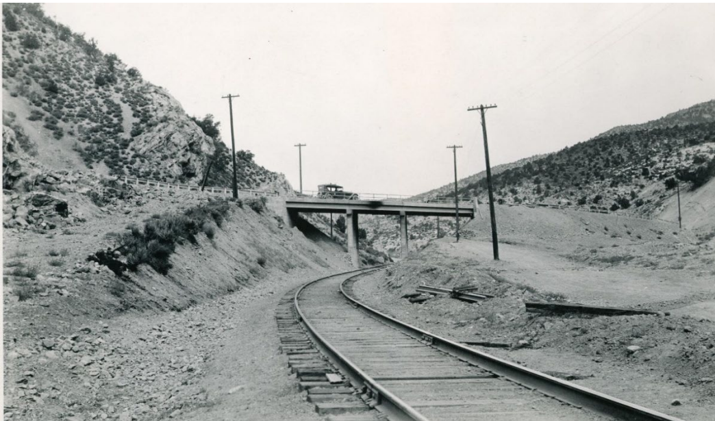
Figure 26. Grade-separation structure one-half mile west of Ely in Robinson Canyon, 1924. 205
