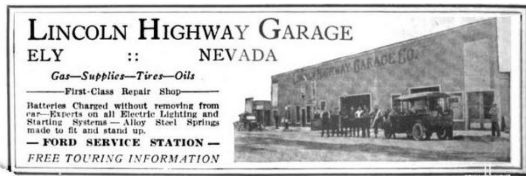
Figure 8. Advertisement for the Lincoln Highway Garage Company in Ely, Nevada, 1923. 67
