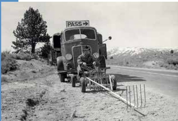
Clear roadway markings save lives
