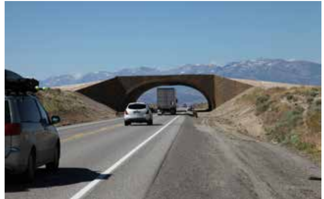
Wildlife and traffic separation for safer travel on roads
