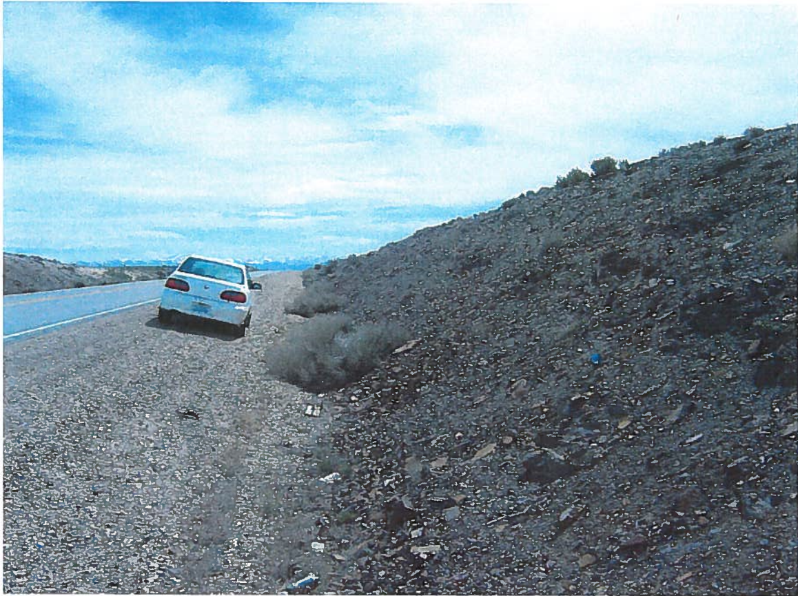
SLOPE # 3 Milepost US93 EL 8+0.7
