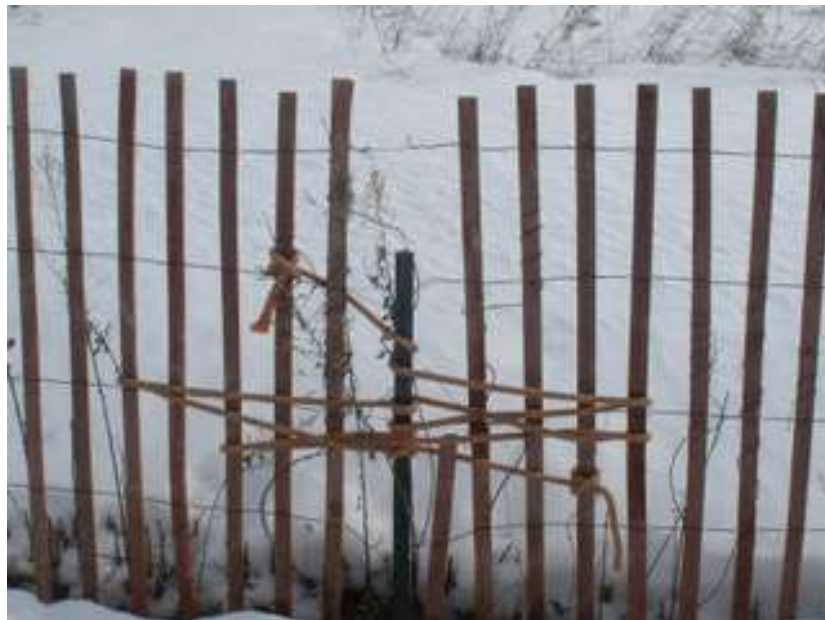
Deteriorated Snow Fence:
