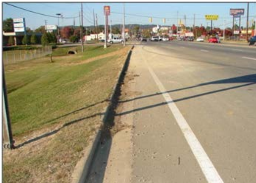
Paved Surface with Accumulated Dirt and Sand:
