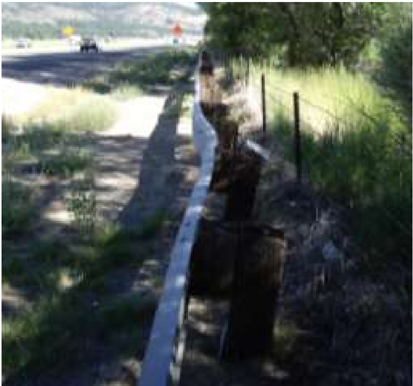
Damaged guardrail:
